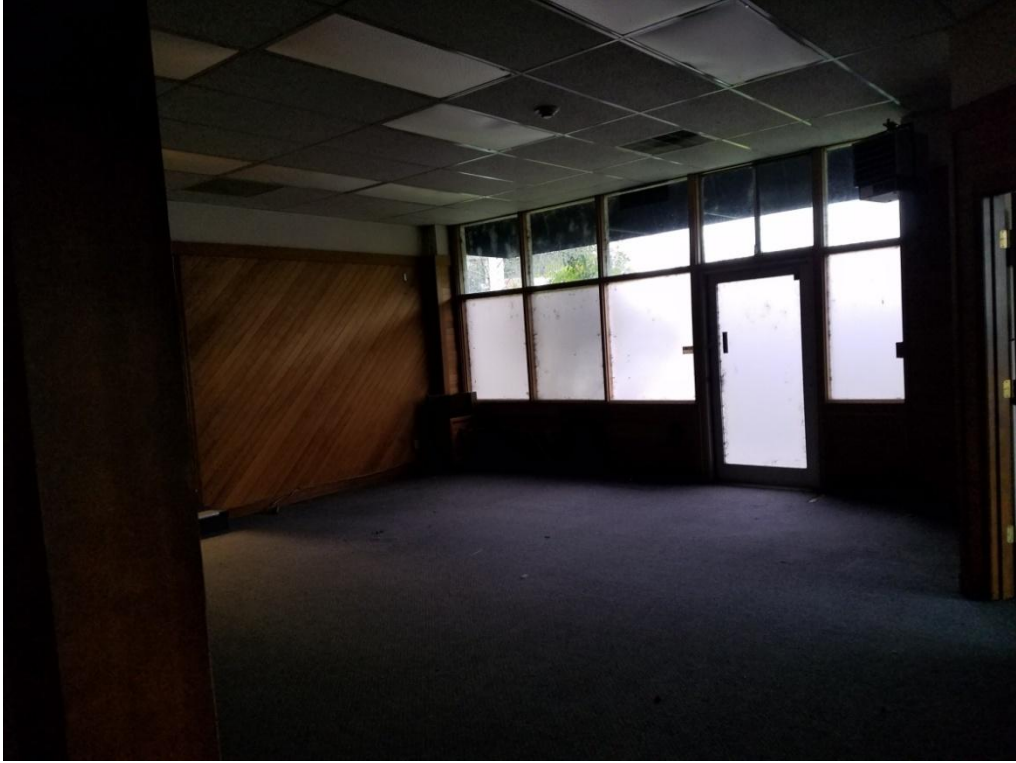
Main Level Interior looking toward Hwy 43
