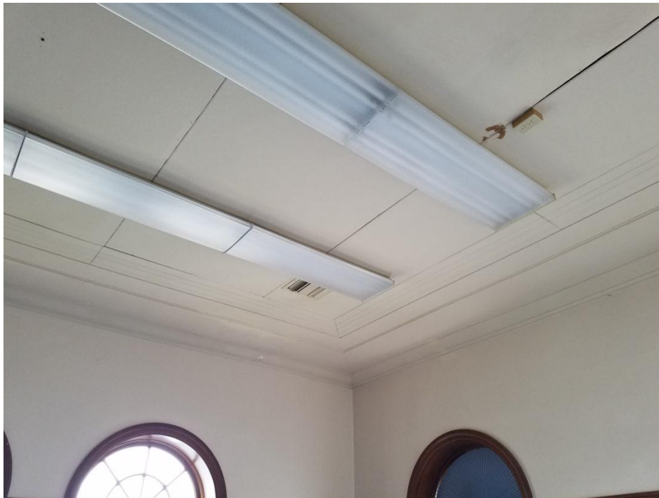
Original Ceiling Detail with existing light fixtures
