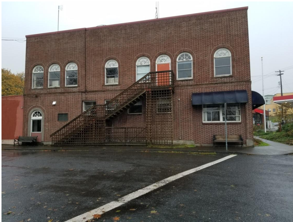
Left side- Mill St facade
