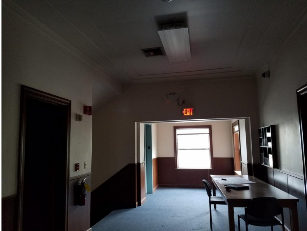
Upper Level Stair/ Elevator Lobby
