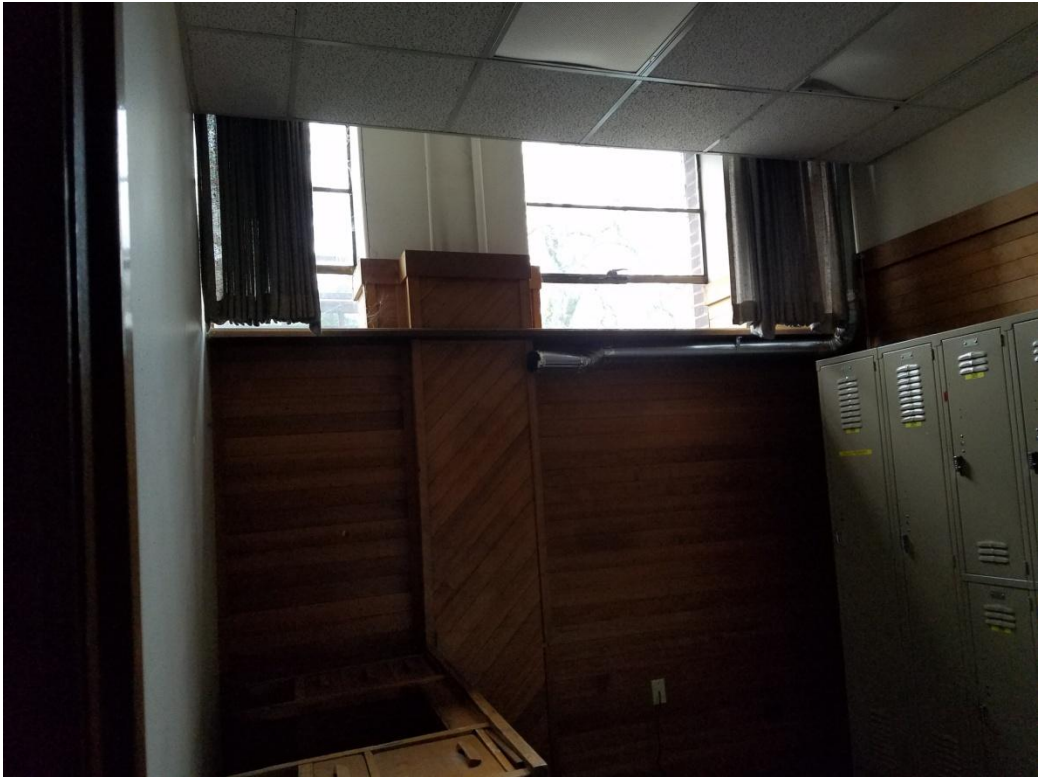
Main Level Offices along Mill St
