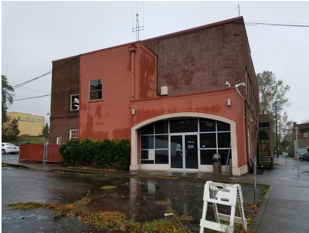
Rear Façade with 1980's addition
