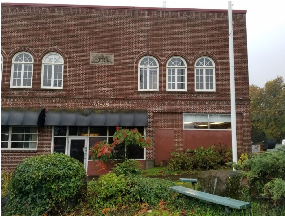
Front façade showing infill areas
