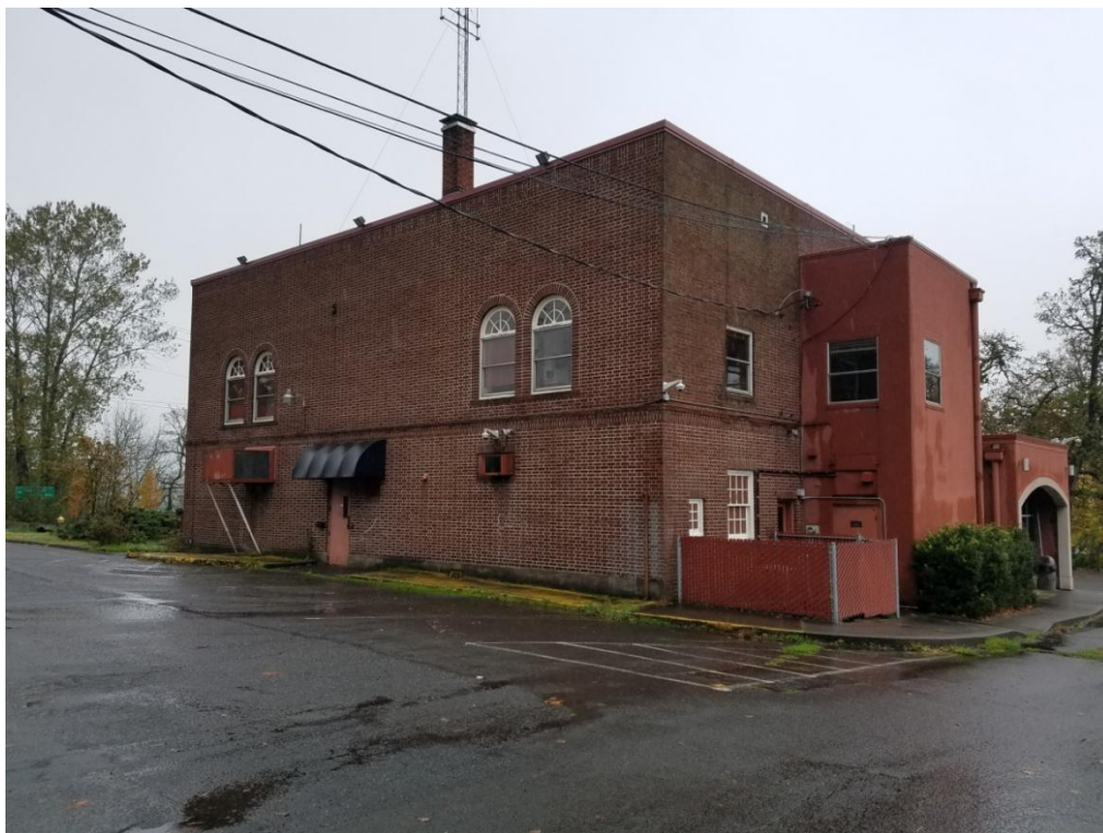
Right and Rear Facades
