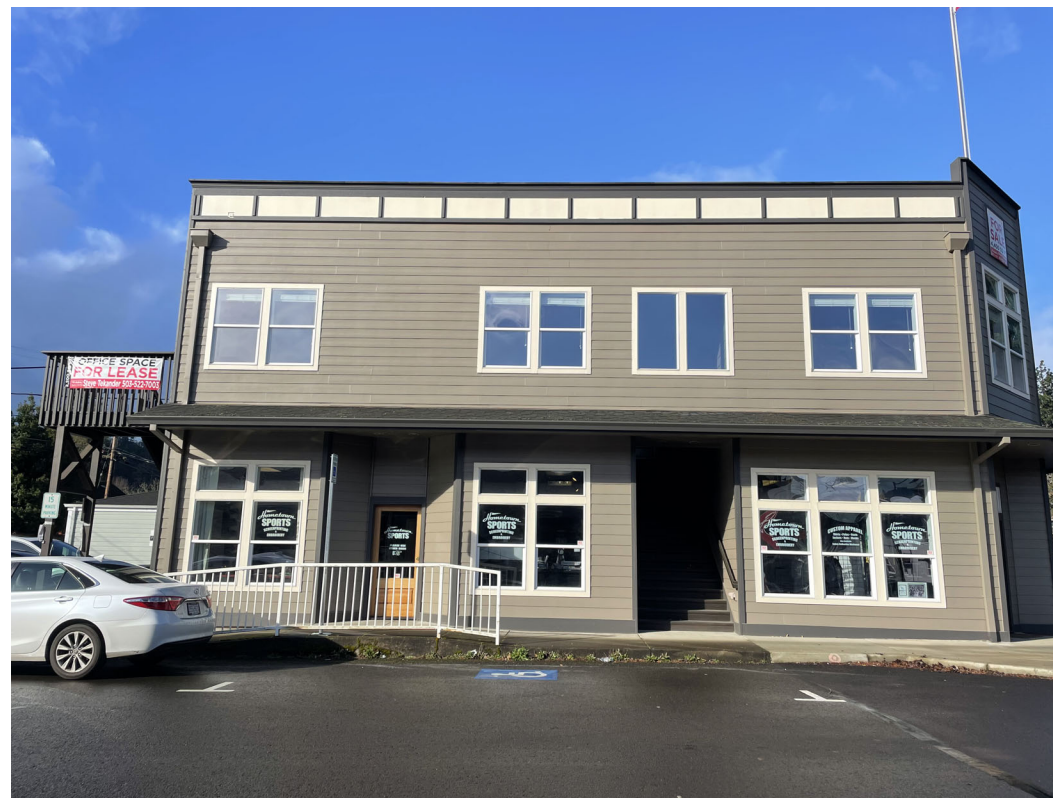
EAST FACADE ALONG 13TH STREET
