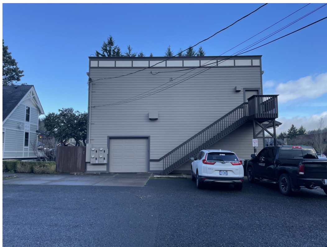
SOUTH FACADE BEHIND BUILDING
