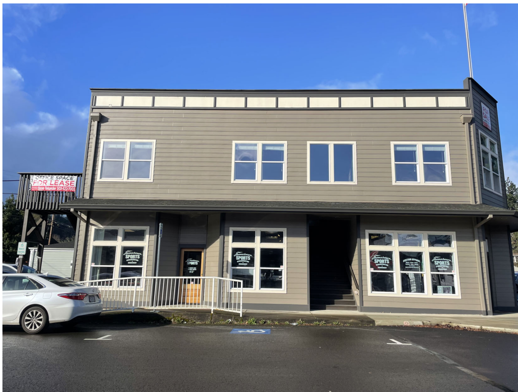
EAST FACADE ALONG 13TH STREET
