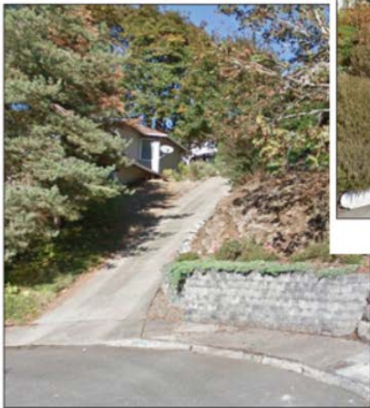
2463 Tipperary Court – 33% driveway grade
