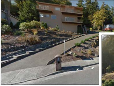
6080 Caufield Drive – 19% driveway grade
