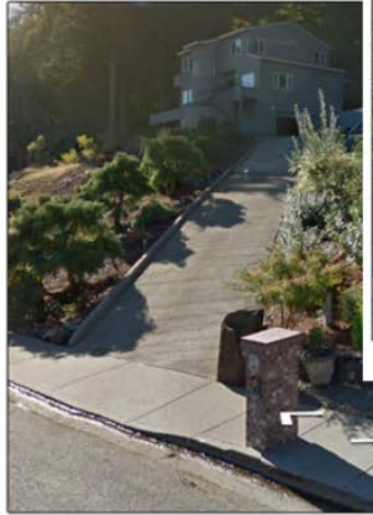
6040 Caufield Drive – 24% driveway grade
