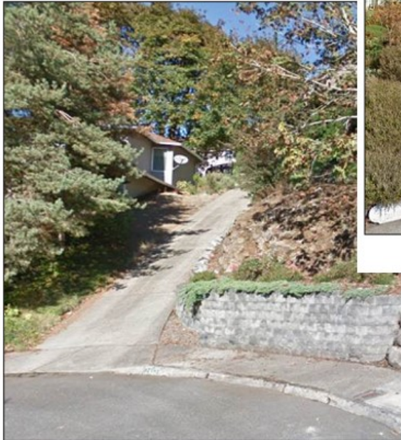
2463 Tipperary Court – 33% driveway grade
