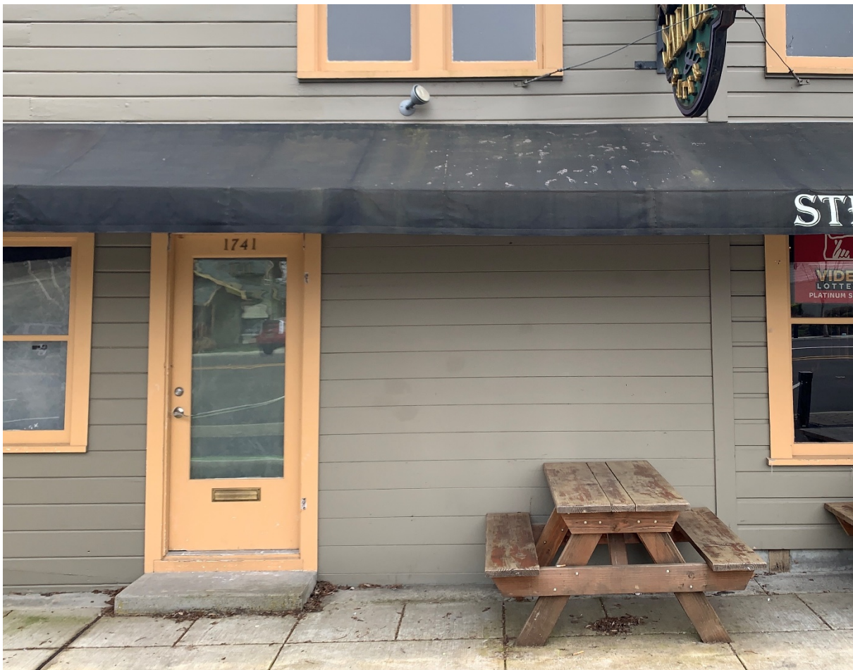
Close-up of existing front façade illustrating the varying horizontal siding patterns on the building.
