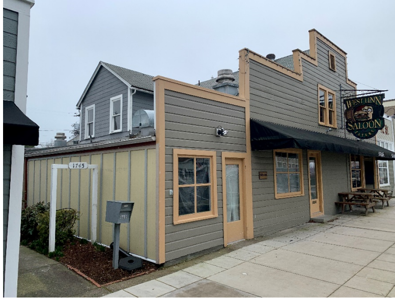
Looking Southeast at building corner.
