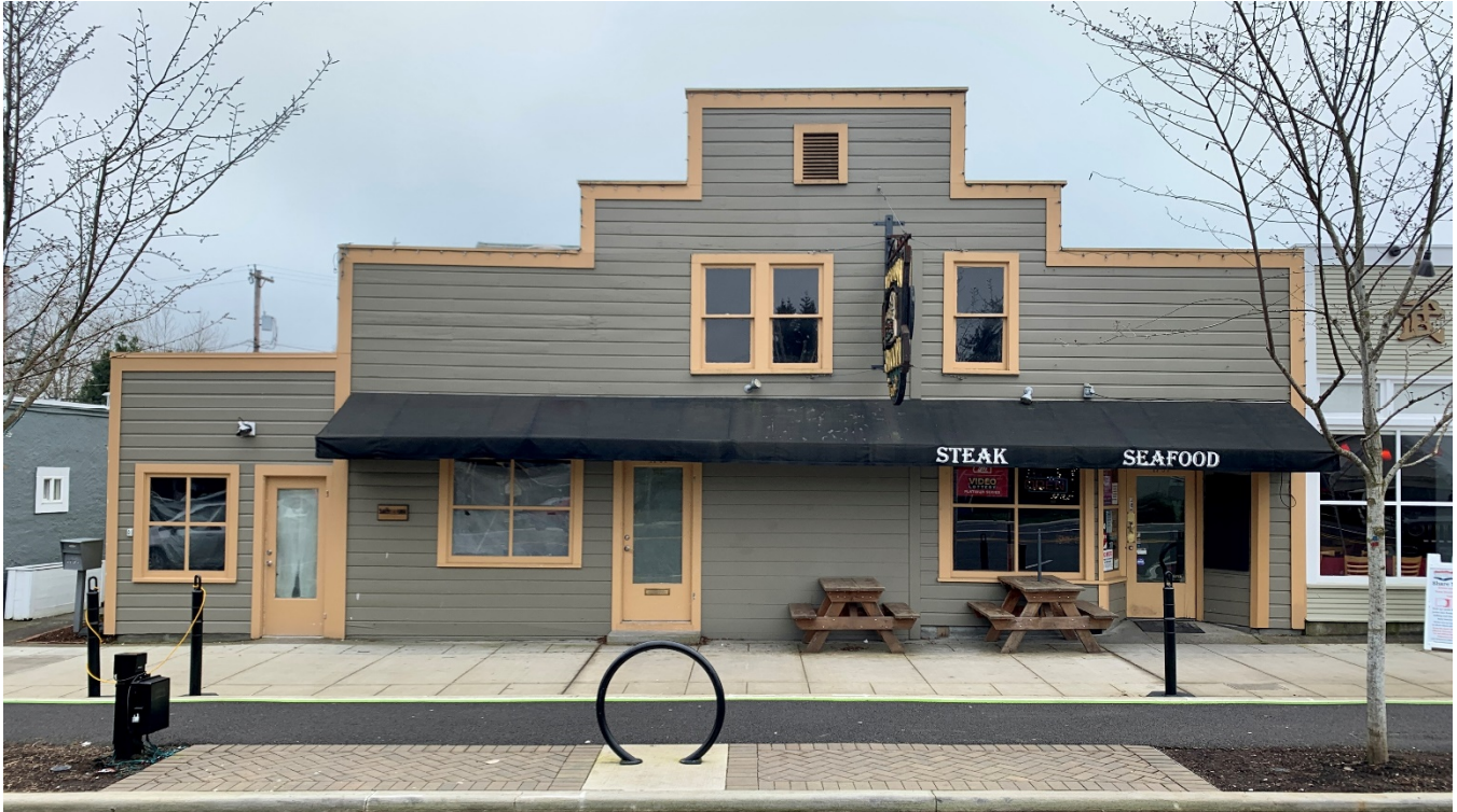
Existing front facade facing Willamette Falls Drive
