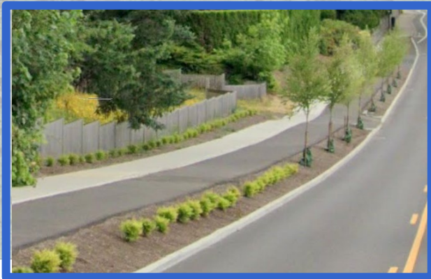
Separated Bicycle Facilities on Willamette Falls Drive
