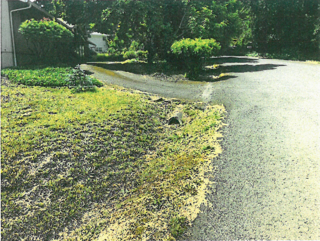
Photo point 1 facing south, southwest at north end of TL 2300
