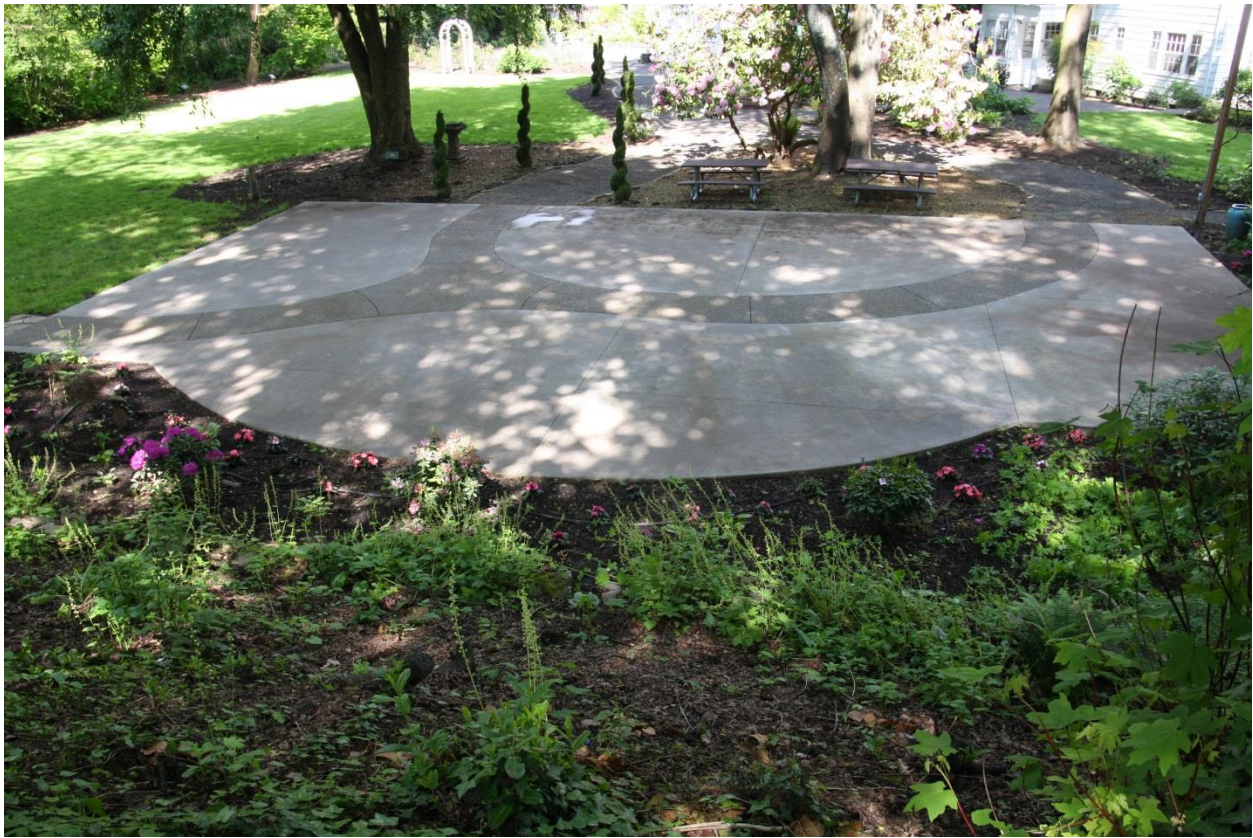
Figure 3: Existing Concrete Slab Image provided by West Linn Parks and Recreation
