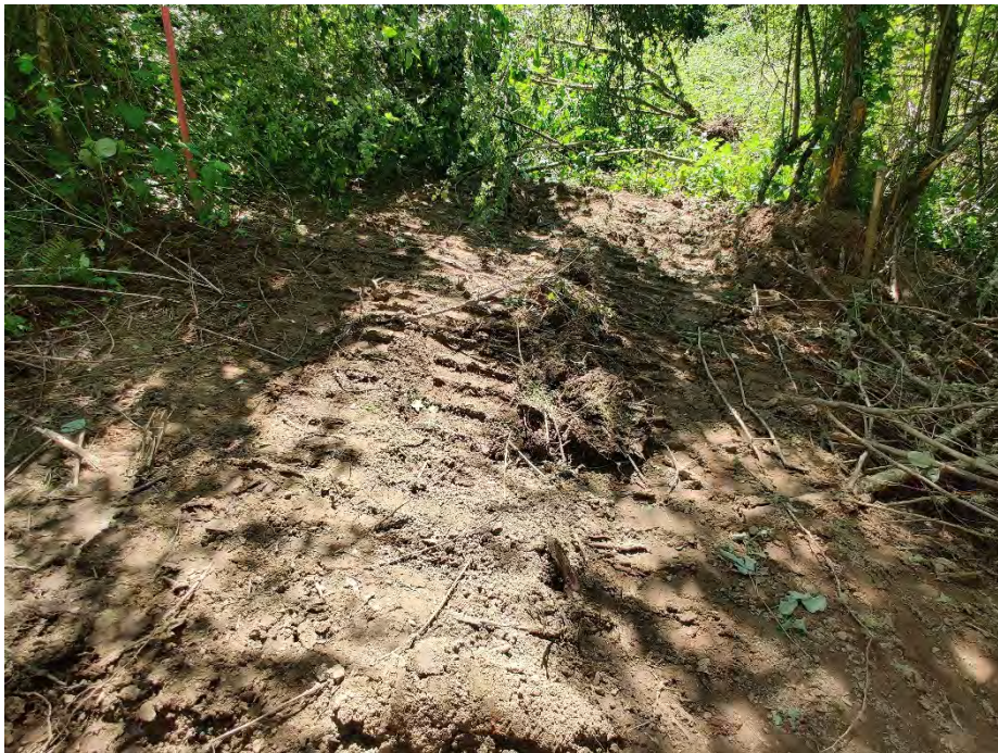
Photo 12. Fresh excavator tracks – western portion of the Site
