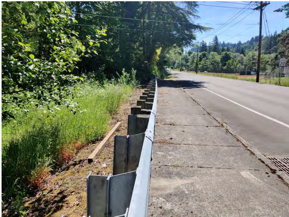
Photo 6. Northwest corner facing southeast
