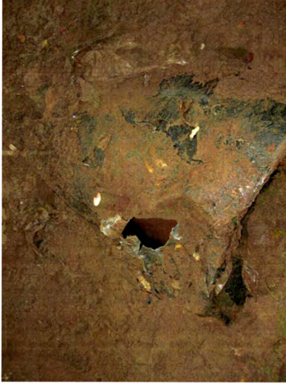
Tank was empty (no product in tank)
