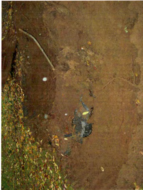
Top of tank
