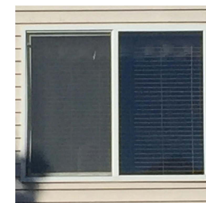
W-1 VINYL WINDOWS 1280 Single-Slider Window (White or Almond to match existing) MI Windows
