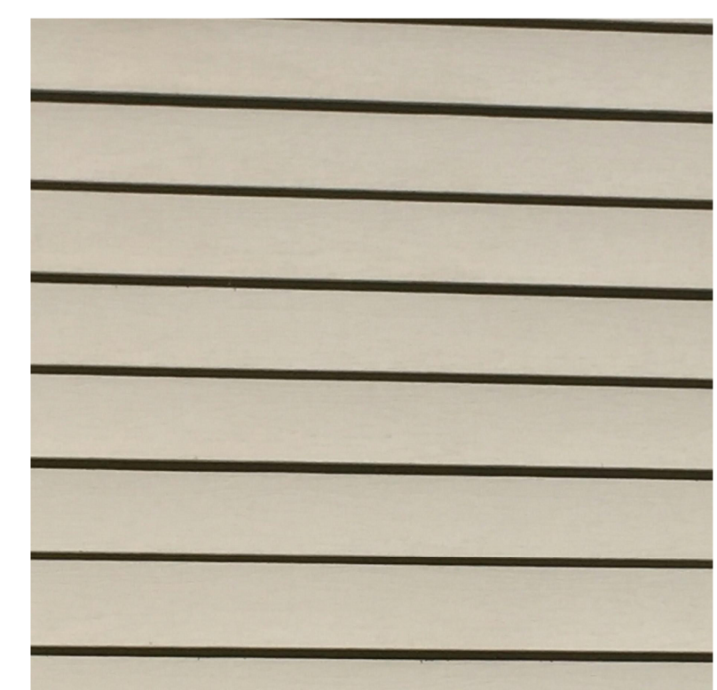
S-1 SIDING Fiber Cement Siding, paint color to match existing vinyl siding
