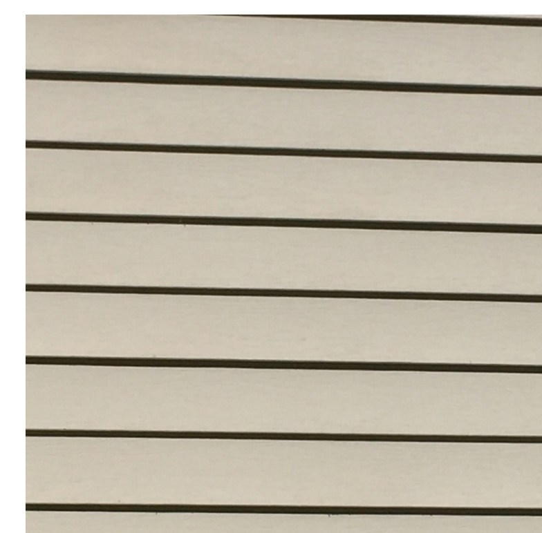
S-1 SIDING Fiber Cement Siding, paint color to match existing vinyl siding
