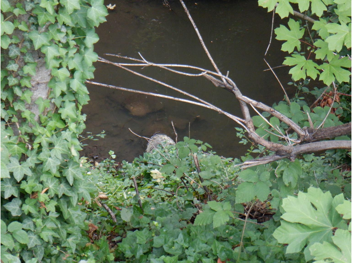
Figure 4. Pipe down existing embankment from site into the Cascade Springs Pond Creek.
