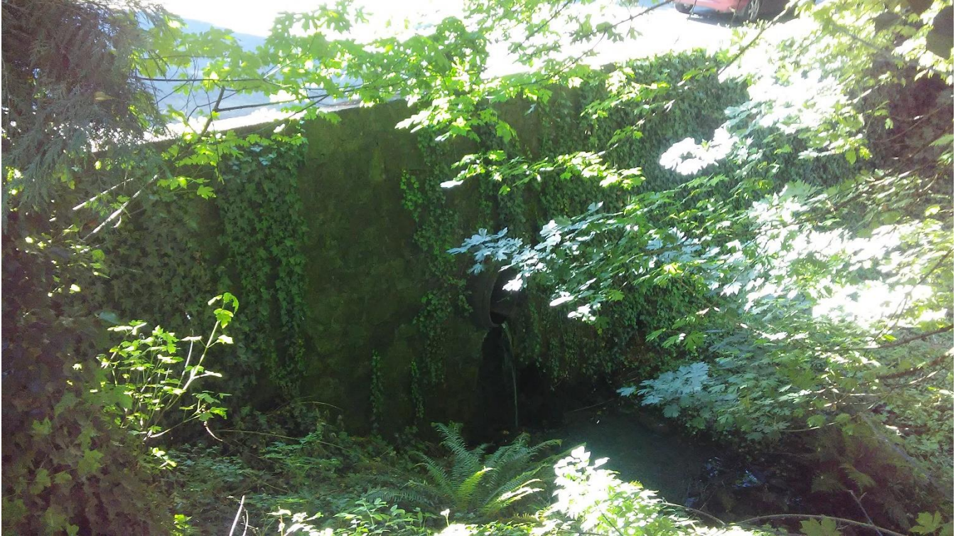
Figure 3. Cascade Springs Pond Creek looking upstream at the projected barrel of the River St. culvert outlet (30" diam).
