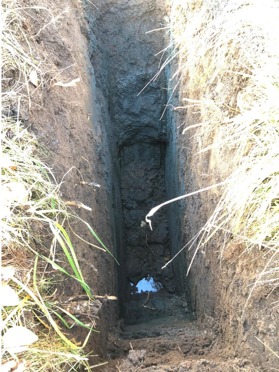
Test Pit TP-1
