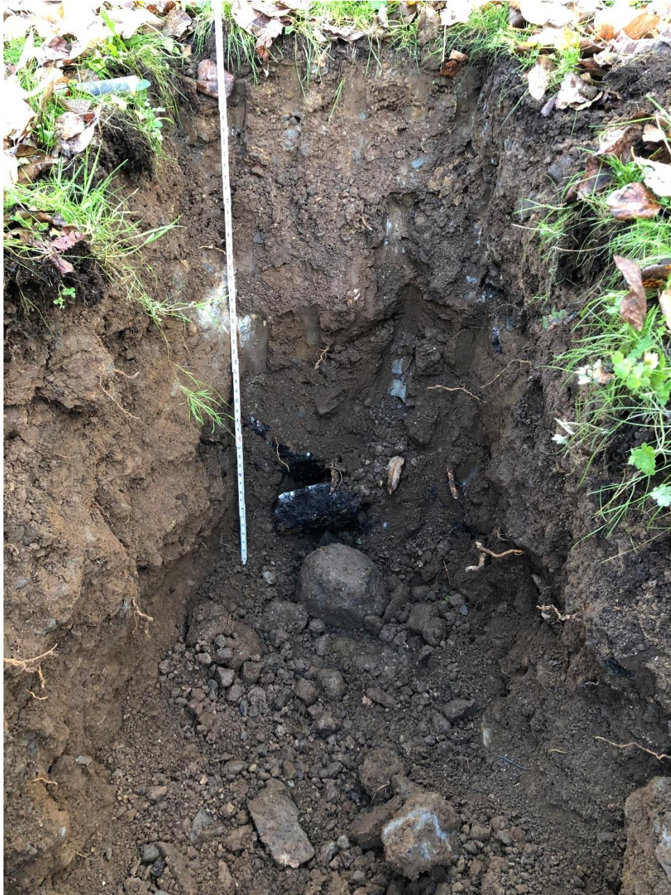
Test Pit TP-1 Undocumented Fill
