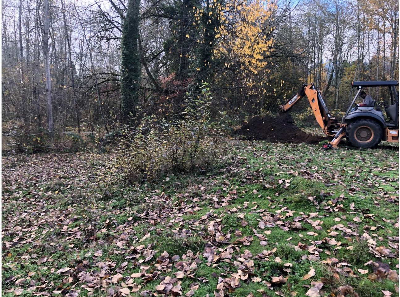
Test Pit TP-3
