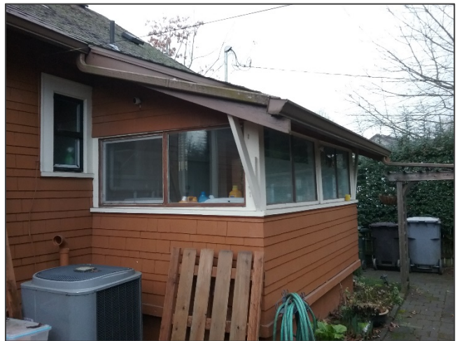
Rear Shed Addition
