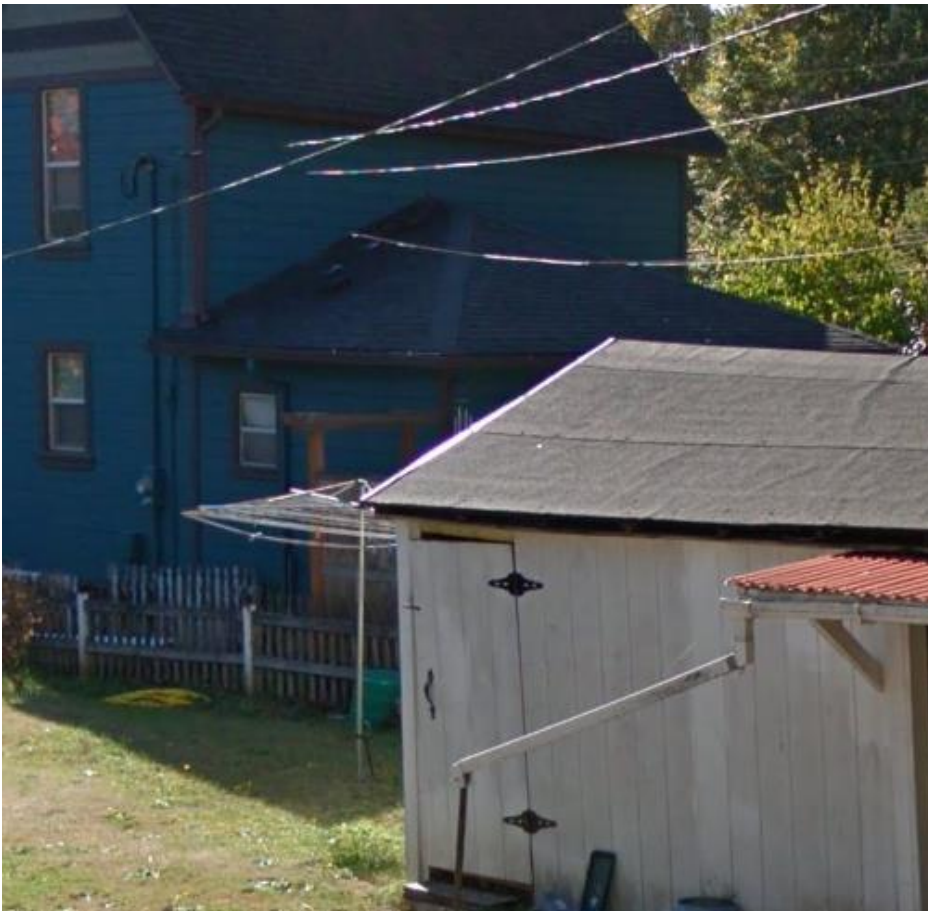
1409 14 th St. - Addition extending from width of original exterior walls.
