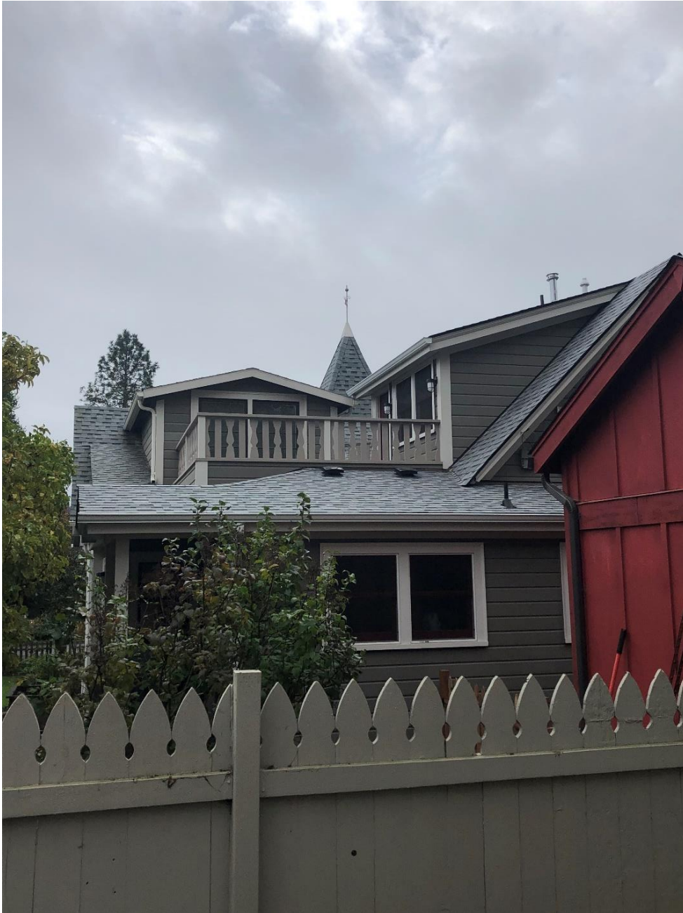
1822 5 th Ave. – 3:12 Gable
