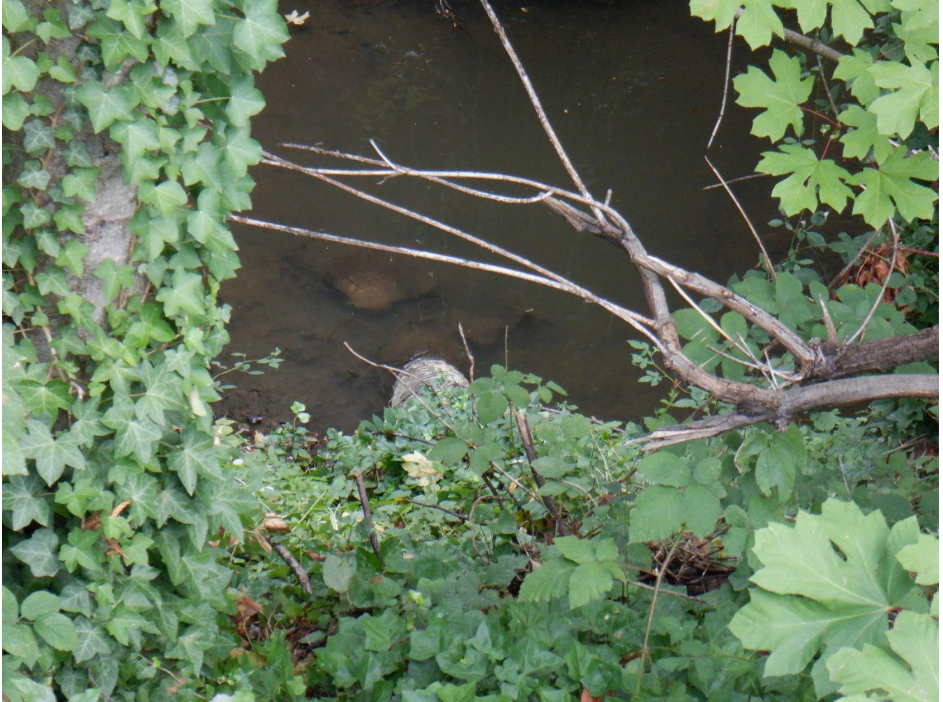
Figure 4. Pipe down existing embankment from site into the Cascade Springs Pond Creek.
