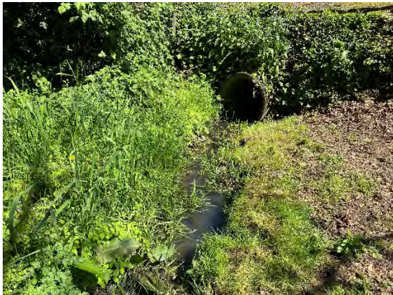
1900 ft downstream looking east
