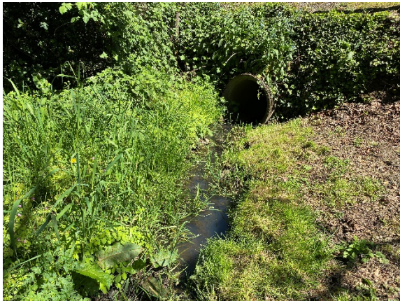
1900 ft downstream looking east
