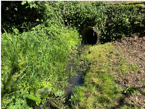
1900 ft downstream looking east
