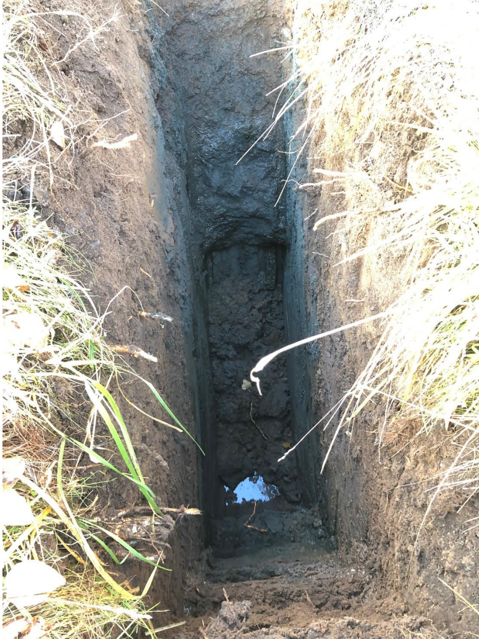
Test Pit TP-1
