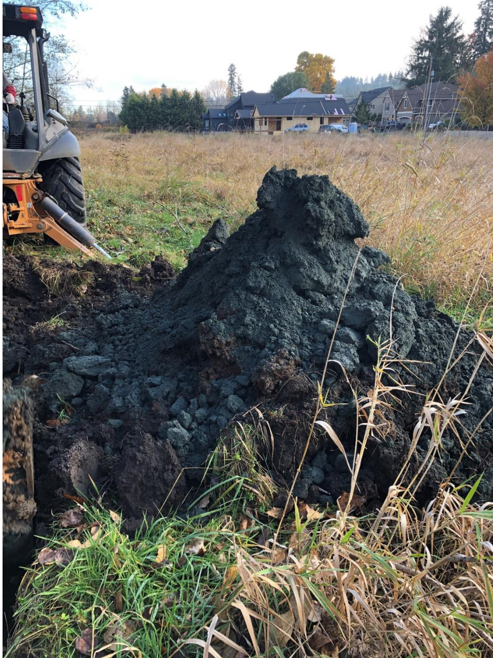
Test Pit TP-4
