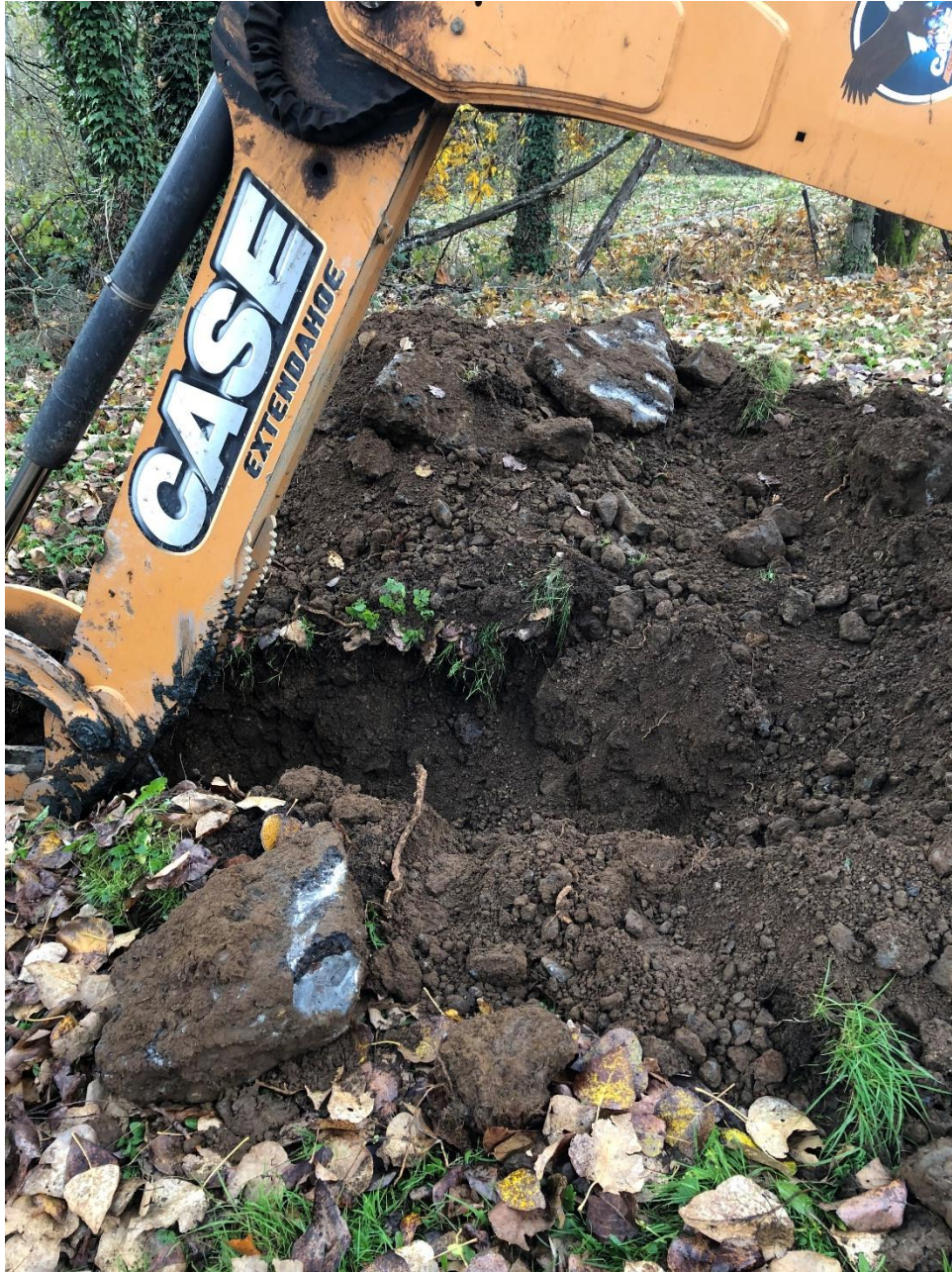
Test Pit TP-2 Undocumented Fill
