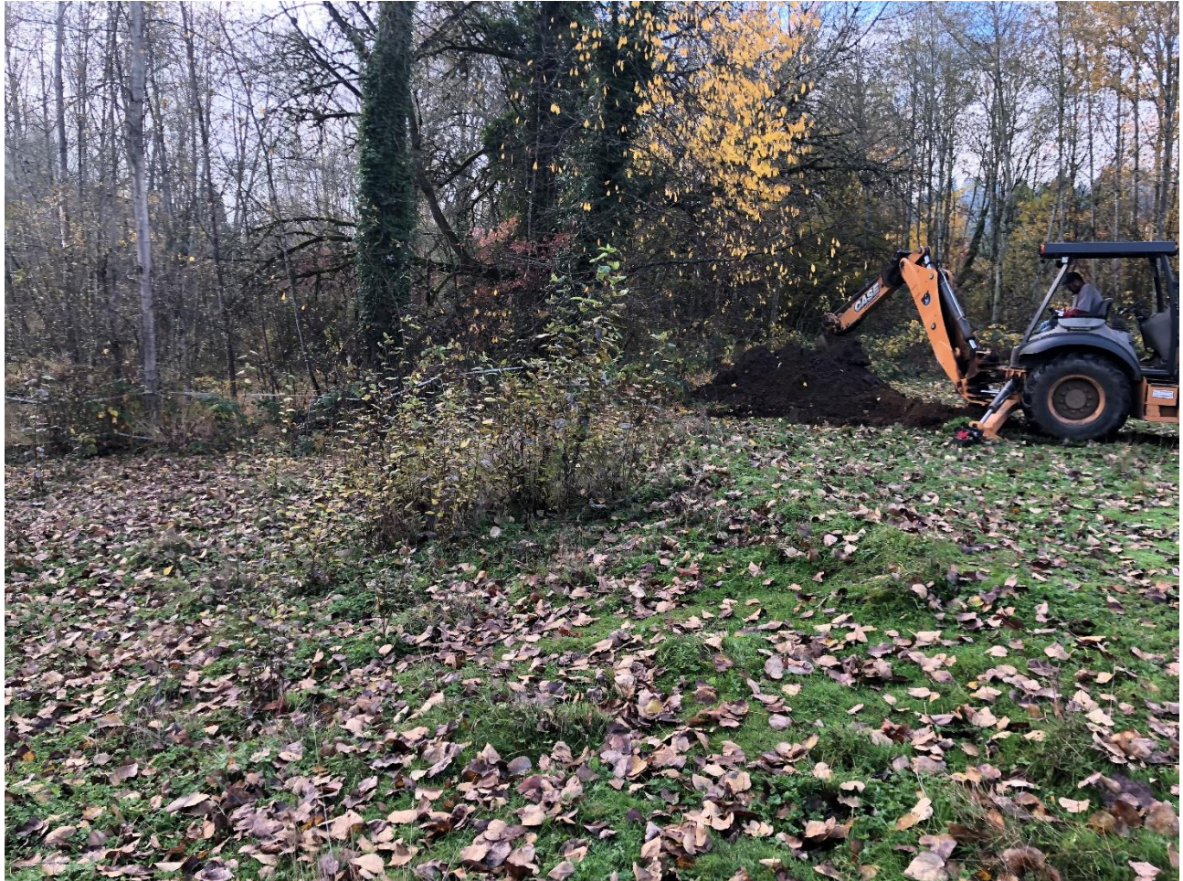
Test Pit TP-3
