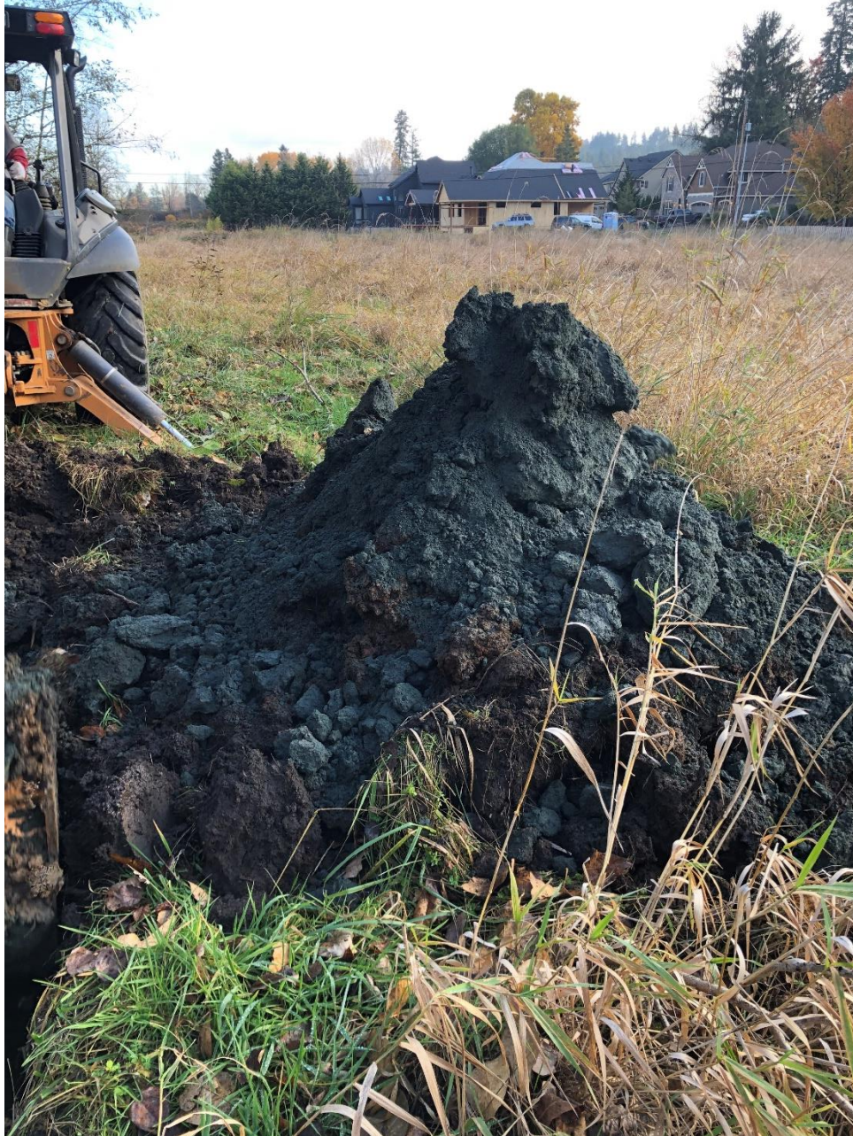
Test Pit TP-4
