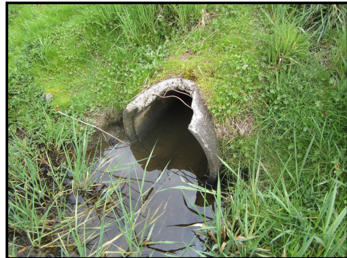
Photo H. 18-inch concrete culvert under 9th Street.
