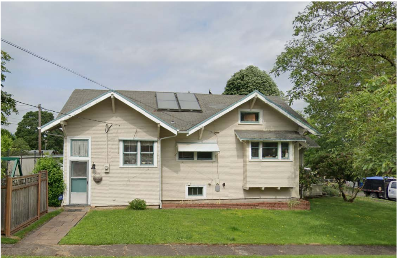
West Elevation (Side – taken from 13 th Street)
