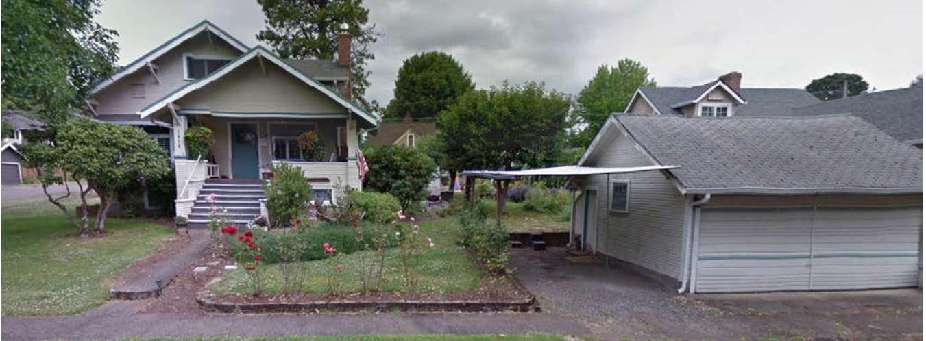
North (Front) Elevation (taken from 4 th Ave)
