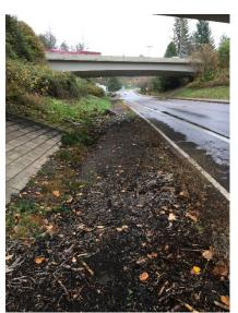
Flat topography and an insufficient stormwater collection system along Blankenship Road frequently results in ponded water and road closures during storms.
