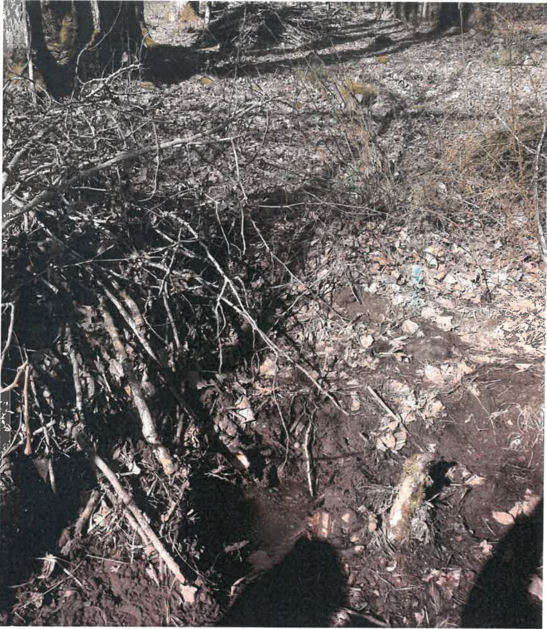
Photo 2. Water seeping from soil in the existing channel into a shallow excavation (bottom center of photo) near the junction of Tannler Drive and Blankenship Road on March 9, 2019. Photo taken looking upstream from near the road junction along the channel axis. The seepage indicates that the channel continues to transmit subsurface water despite the disconnection of the channel from upstream runoff.
