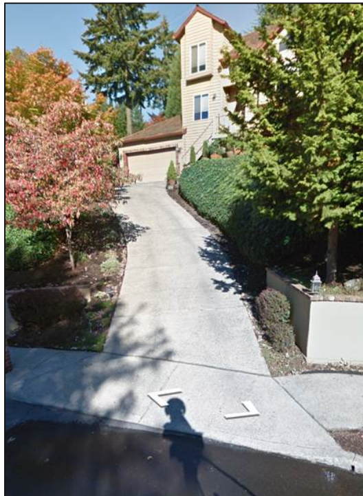
2567 Kilkenny Court – 27% driveway grade
