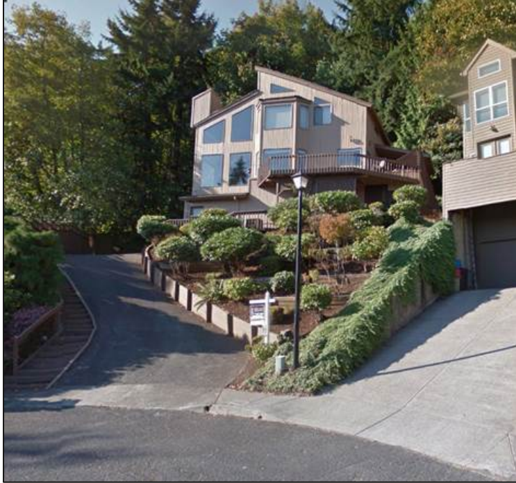
3156 Oak Tree Court – 28% driveway grade
