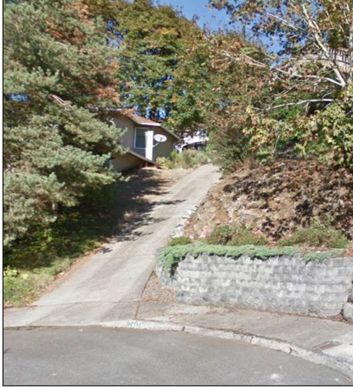
2463 Tipperary Court – 33% driveway grade
