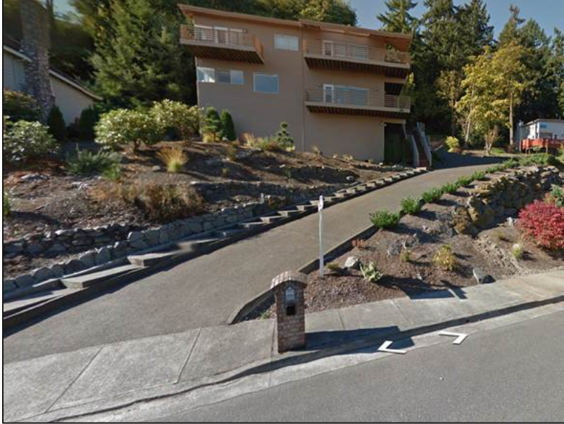
6080 Caufield Drive – 19% driveway grade
