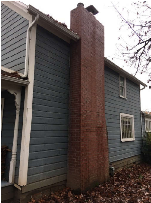
EXISTING RIGHT SIDE VIEW / CHIMNEY
