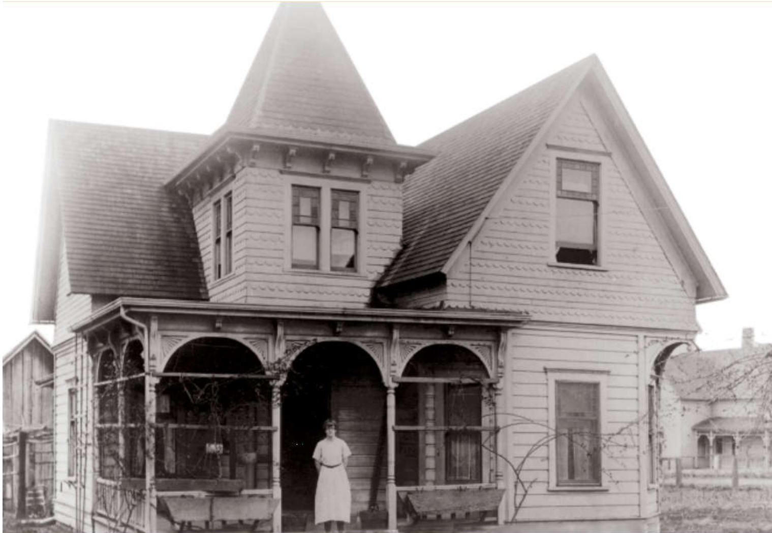
The Joseph H. Ralston House, ca 1910. See No. 30 on the tour.
