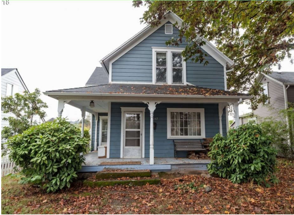
EXISTING FRONT VIEW FROM 6th AVENUE
