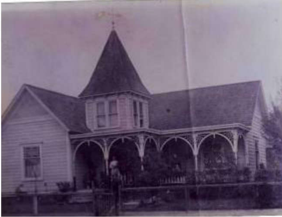
1822 5 th Ave- Miller-Baker House (1899)
