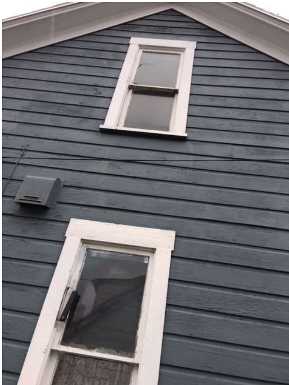
EXISTING WINDOWS / TRIM
