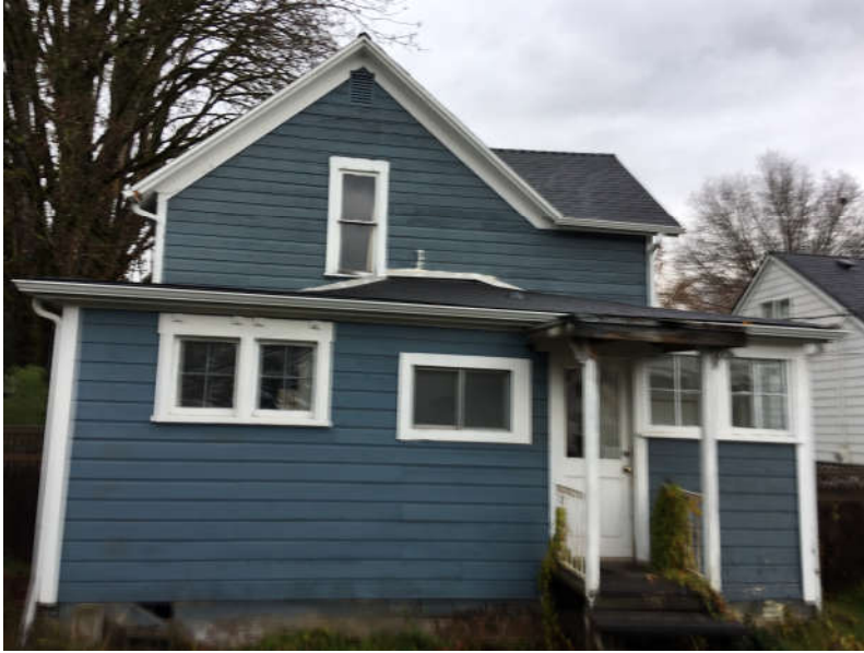
EXISTING REAR VIEW FROM ALLEY
