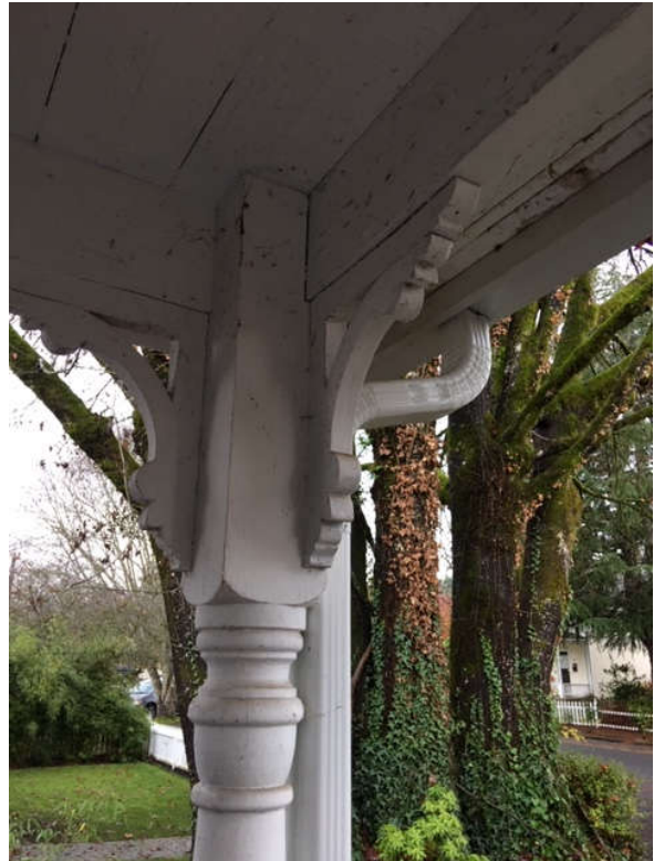
EXISTING FRONT PORCH POST DETAIL
