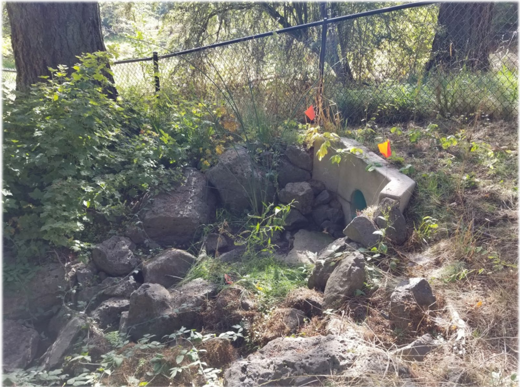
Photo Point 3. Facing southeast toward culvert.
