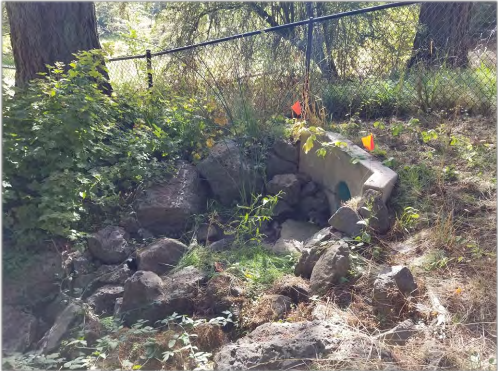
Photo Point 3. Facing southeast toward culvert.
