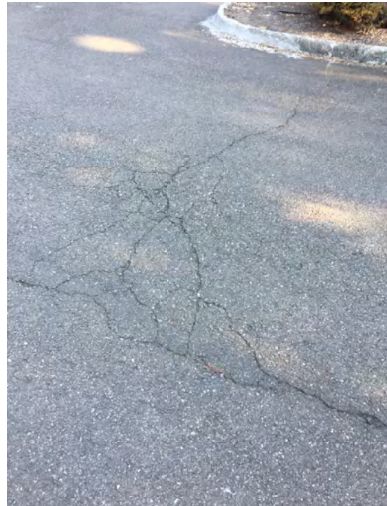
Photograph 4: Fatigue Cracking
