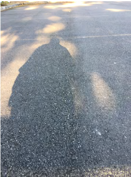
Photograph 3: Surface Raveling
