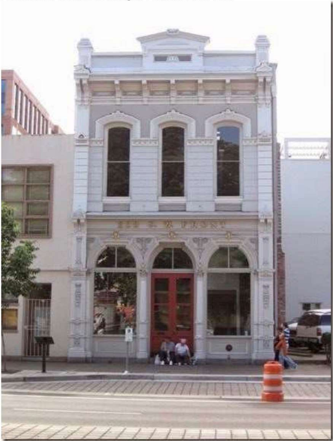
Fechheimer & White Building in Portland circa 1883
