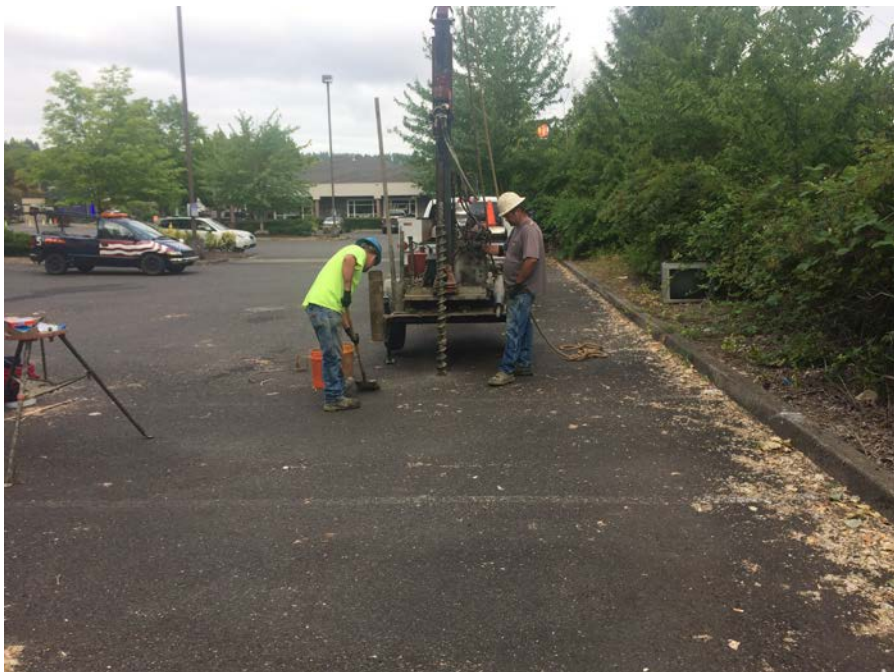
Boring B-1, Facing West
