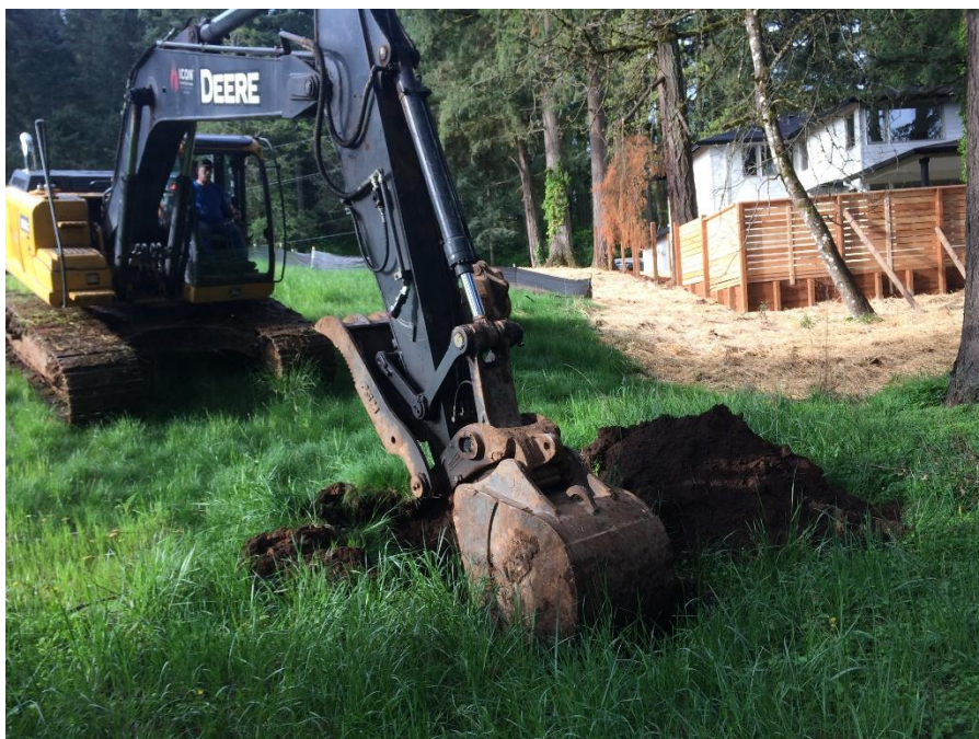
Test Pit TP-1, View of Property Facing South
