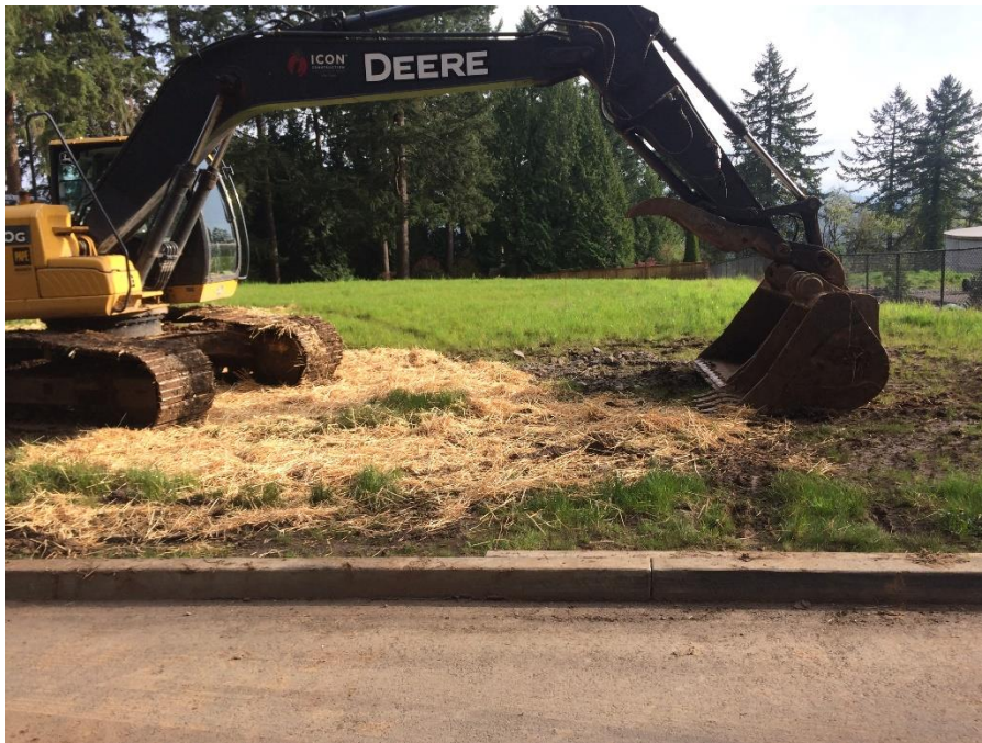
View of Property Facing North
