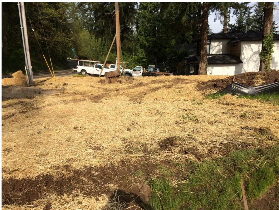
South Side of Property Where House was Demolished
