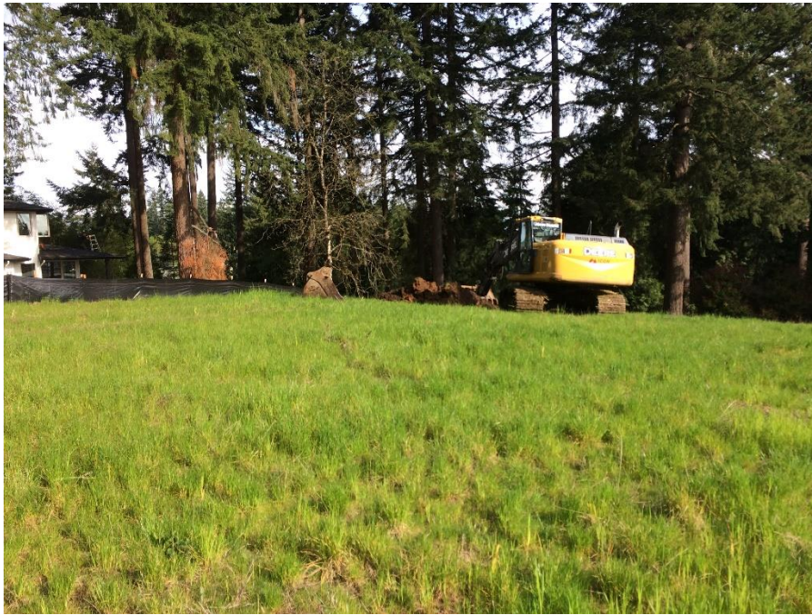
View of Site Facing North
