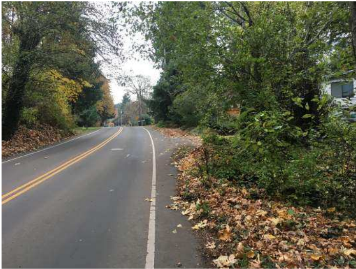
FIG-4A Old River Road facing South approximately 14 feet above existing 36 inch culvert. Steep road slopes of approximately 4-8% toward the culvert crossing based on GIS maps.
