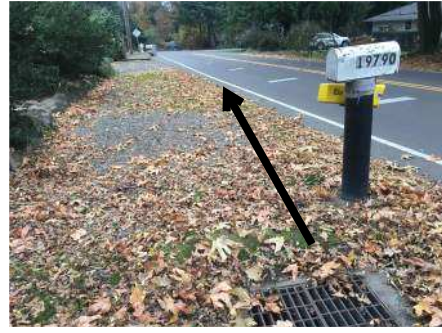
FIG-1 Existing catch basin in Old River Road downstream of proposed Marylhurst School site. 12 inch concrete pipe conveys to the North toward creek. 12 inch concrete pipe 1.9 feet below rim.
