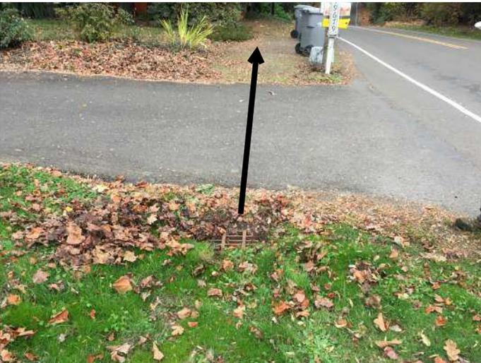
FIG-3 Existing rectangular area drain found approximately 121 LF from circular area drain. Note that rim is approximately 6 inches below adjacent pavement grade. 12 inch concrete pipe found 16 inches below rim grade. Pipe continues North. GIS Map shows an additional area drain/catch basin, but was not found during the site visit.
