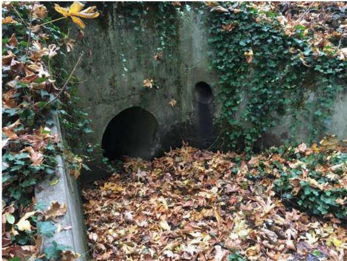
FIG-4B 36 inch culvert and headwalls on the West side of Old River Road. 12 inch outfall is in the headwall to the right of the culvert. Though there are many leaves in the culvert, there does not appear to be any sign of drainage issues at the outfall or culvert. Dense brush and thorned bushes prevent continuation of the analysis downstream of culvert.
