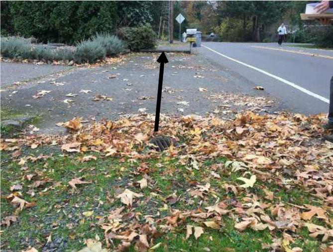
FIG-2 Existing circular area drain in Old River Road. Approximately 62 LF from catch basin. 12 inch concrete pipe found 1.9 feet below rim. Note that GIS maps note a drain where the mail boxes are. No drain was found. Road slopes vary between 2-5% per survey data.
