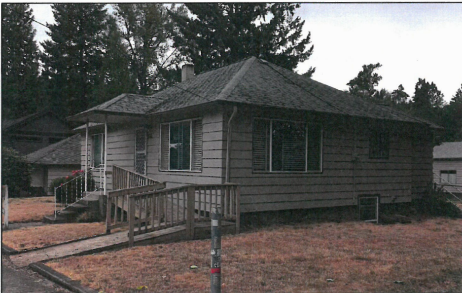
FRONT / SIDE ELEVATION - SOUTHWEST CORNER Street View at Alley Side of Home
