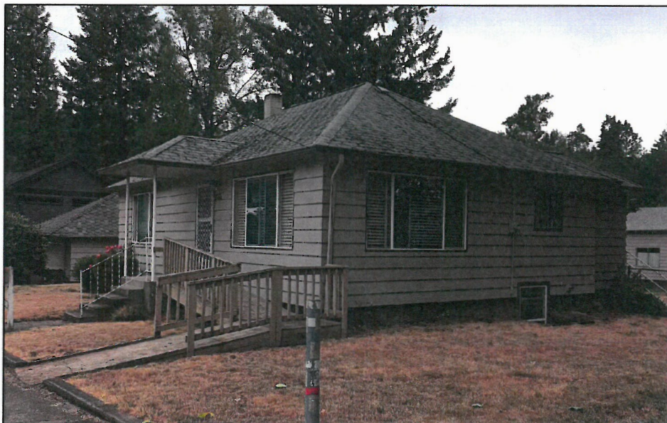
FRONT / SIDE ELEVATION - SOUTHWEST CORNER Street View at Alley Side of Home
