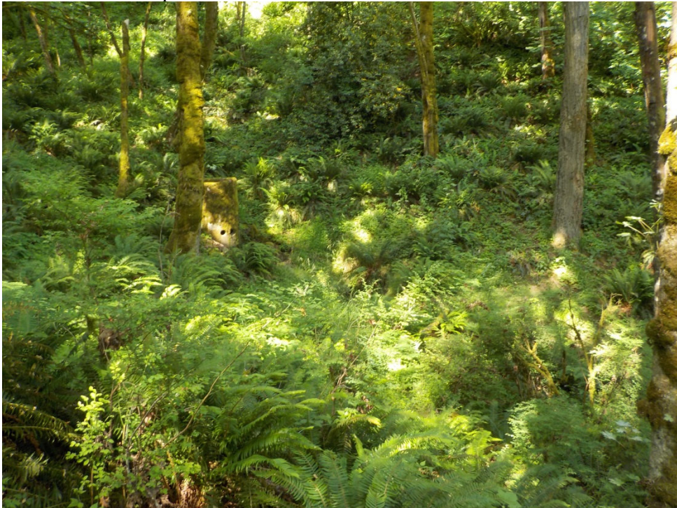
Photo 6 – View of concrete stormwater outflow structure at head of the creek near the site.
