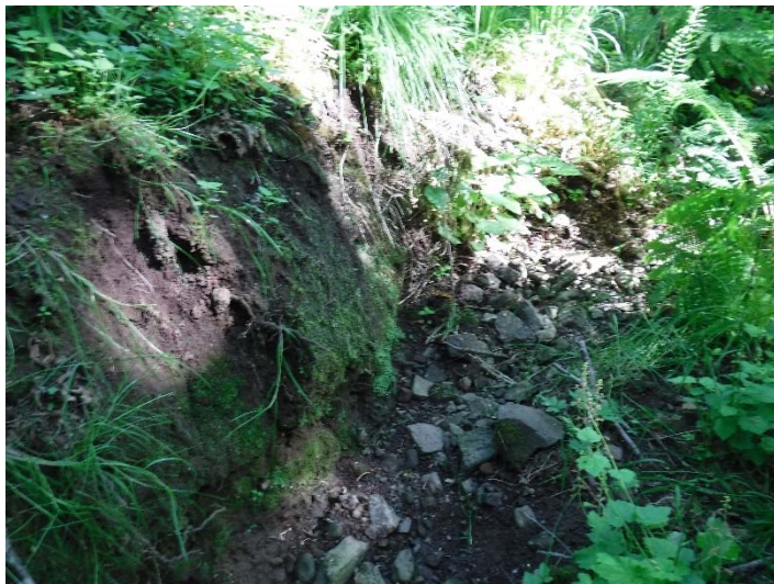
Photo B. View of on site portion of drainage.
