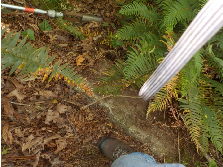
Photo 10 – Close-up view of weathered and partially buried concrete blocks observed near the southern portion of the site.
