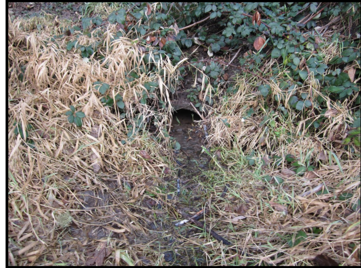
Photo B. View west of buried 12 inch concrete pipe draining stormwater from north into wetland.
