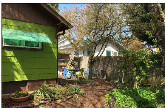
FRONT ELEVATION - SOUTH Looking Toward East Side Yard
