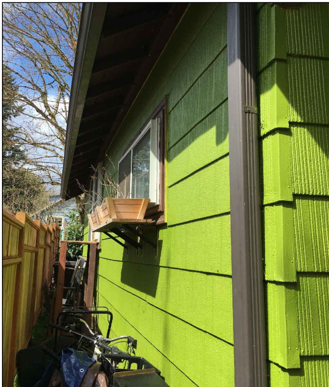
SIDE ELEVATION - WEST View Along West Fenceline
