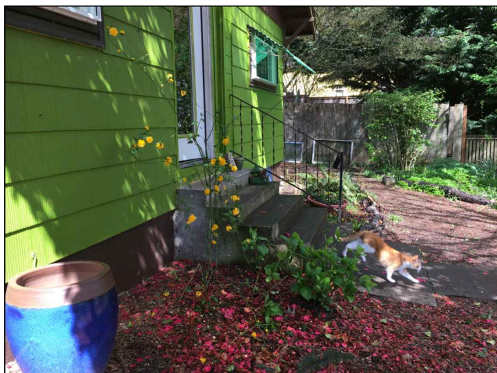
FRONT ELEVATION - SOUTH Detail of Concrete Steps
