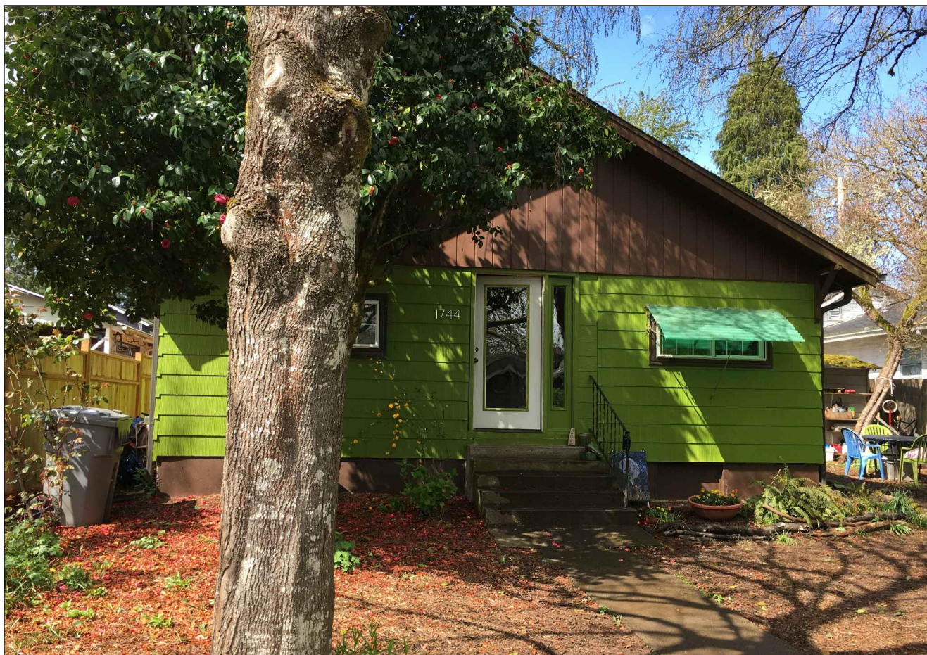
FRONT ELEVATION - SOUTH Street View From Sidewalk
