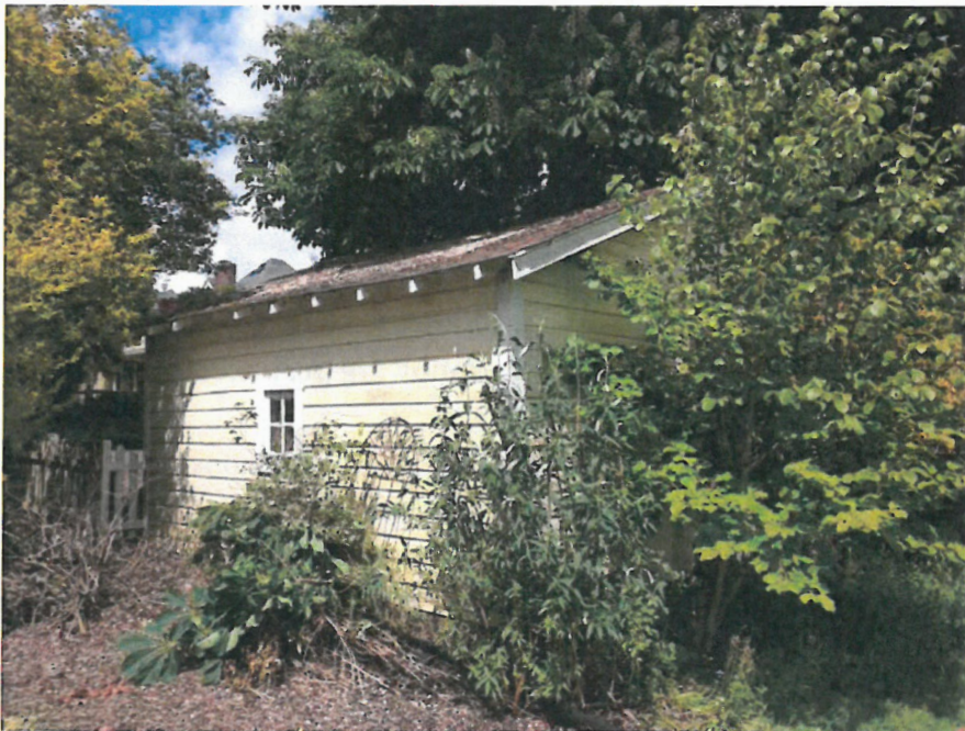
Existing Garage from the Southwest
