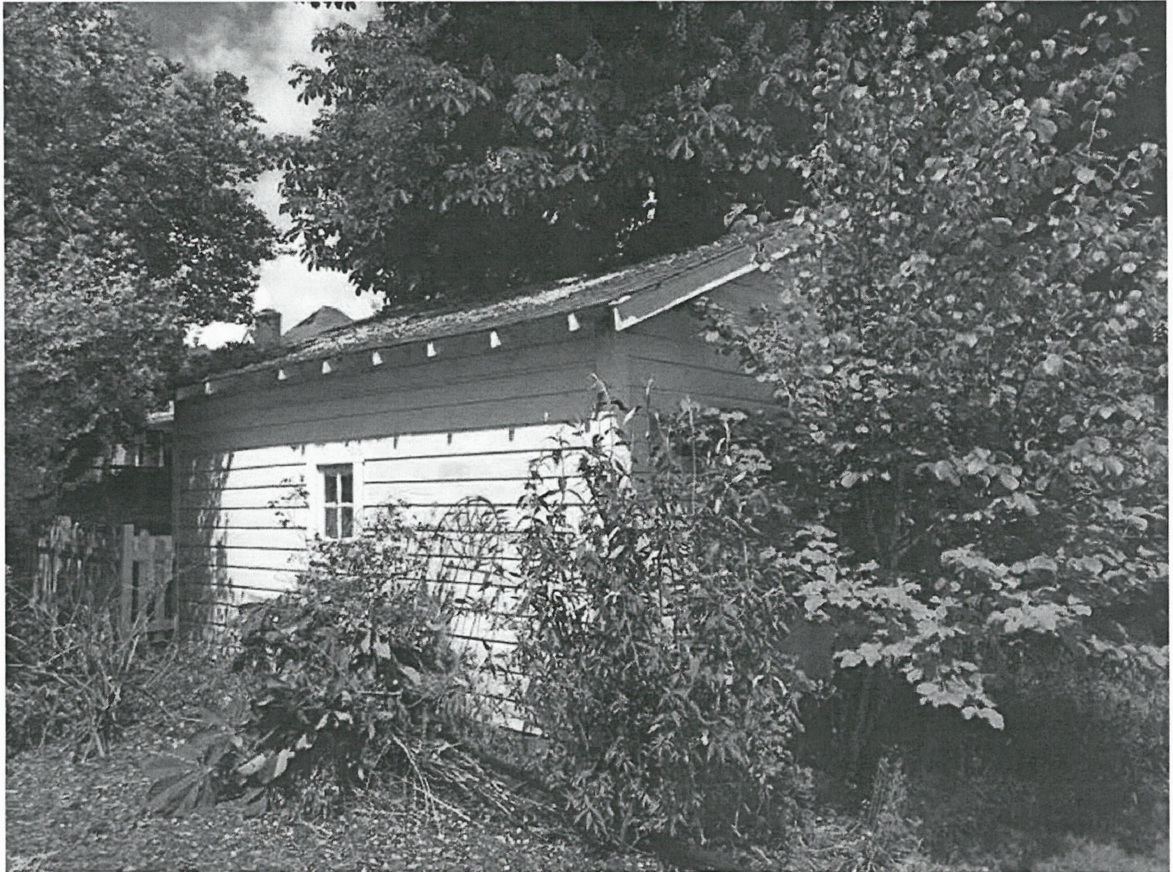
Existing Garage from the Southwest
