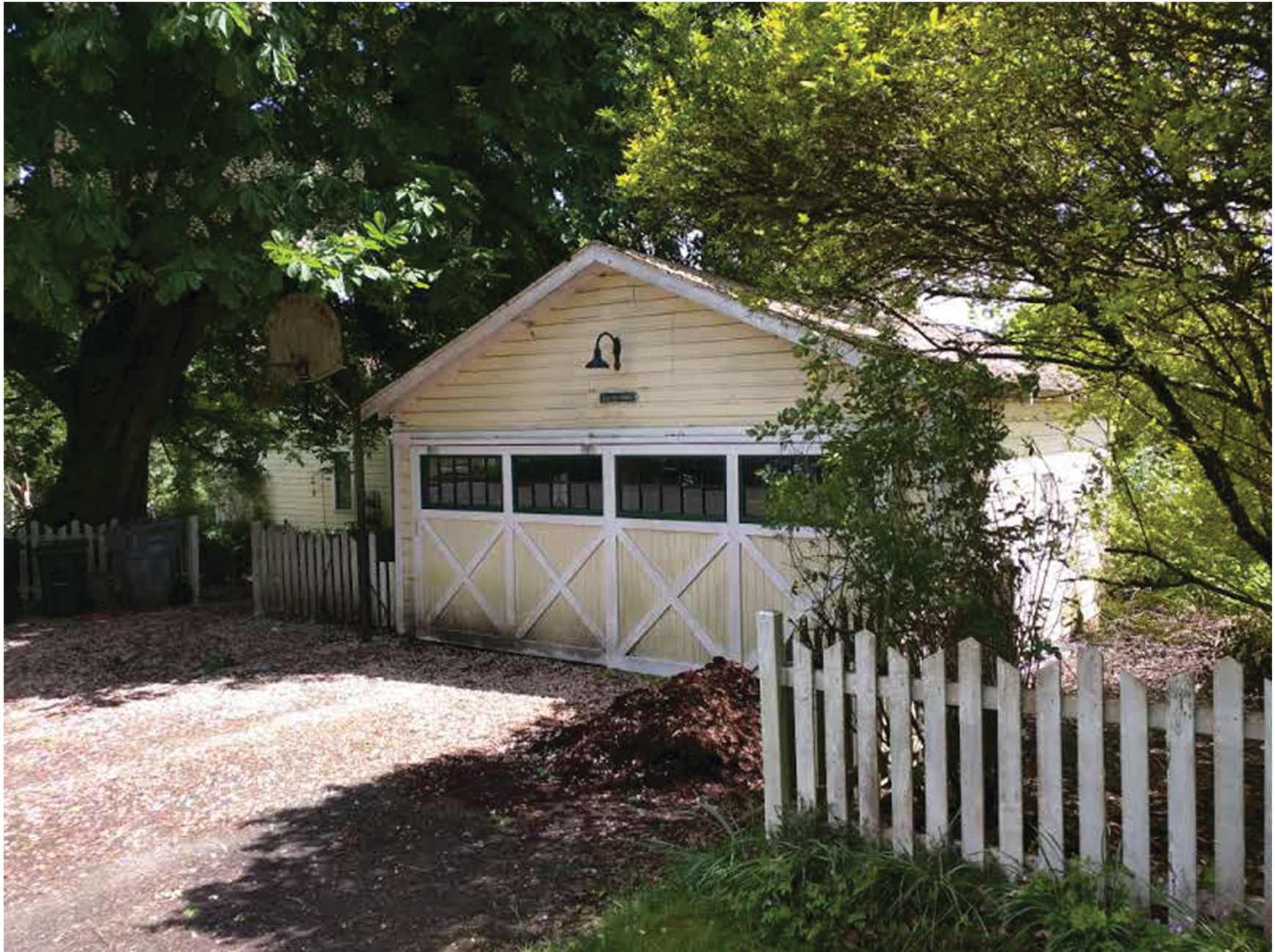
Existing Garage from the Northwest
