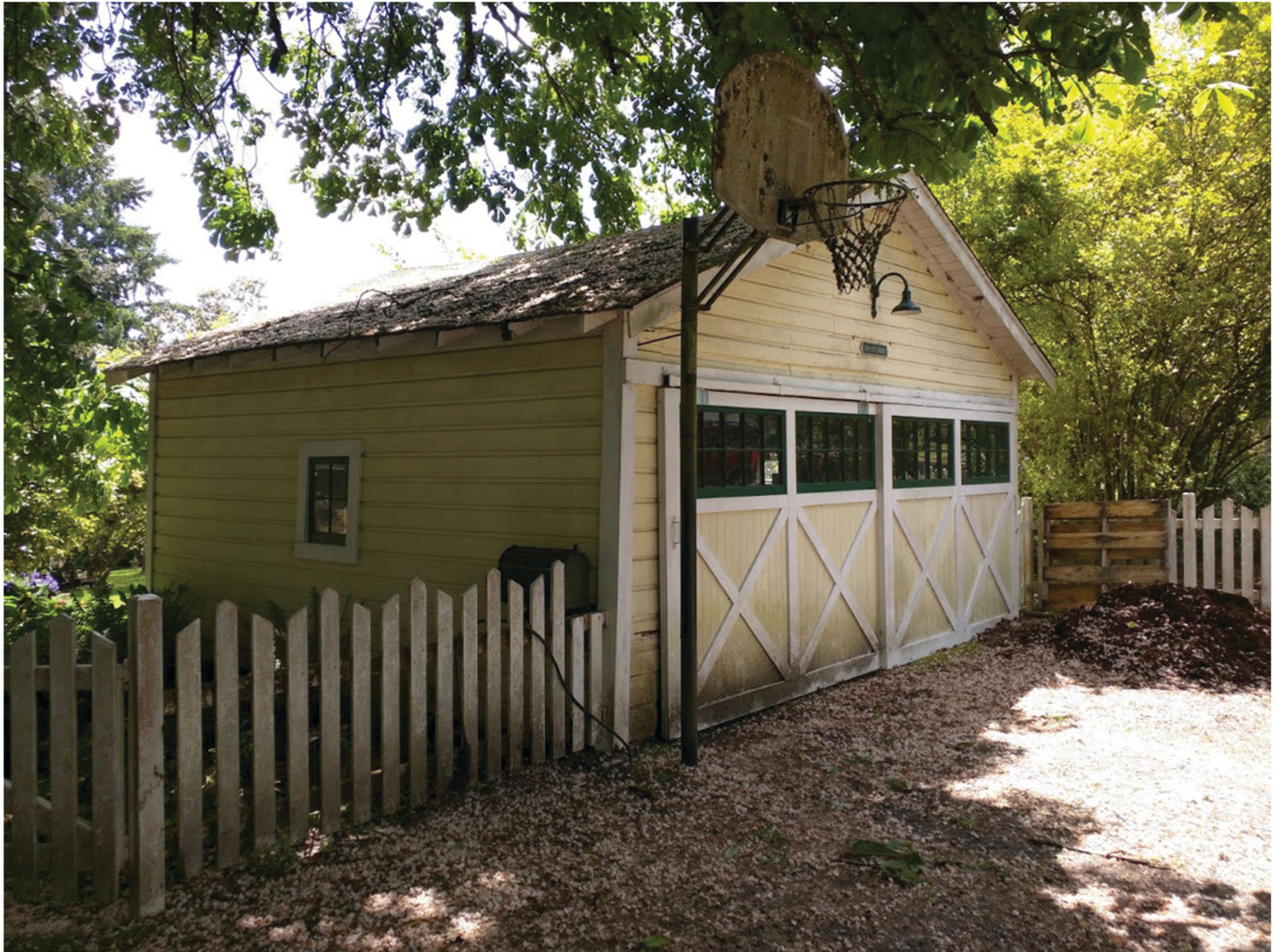
Existing Garage from the Northeast
