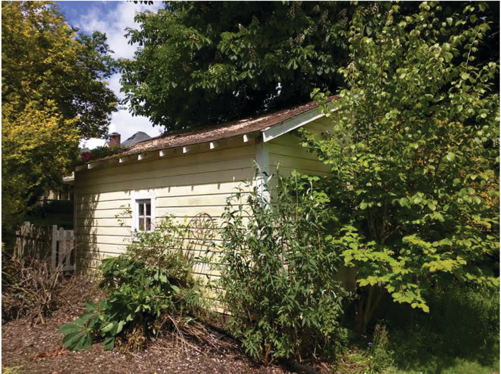
Existing Garage from the Southwest
