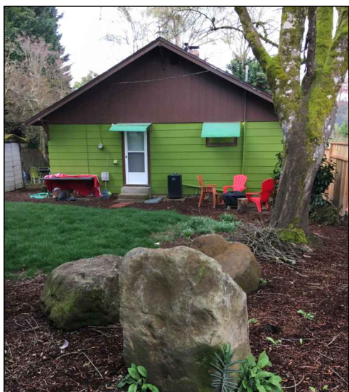
REAR ELEVATION - NORTH View From Alley Along West Fenceline
