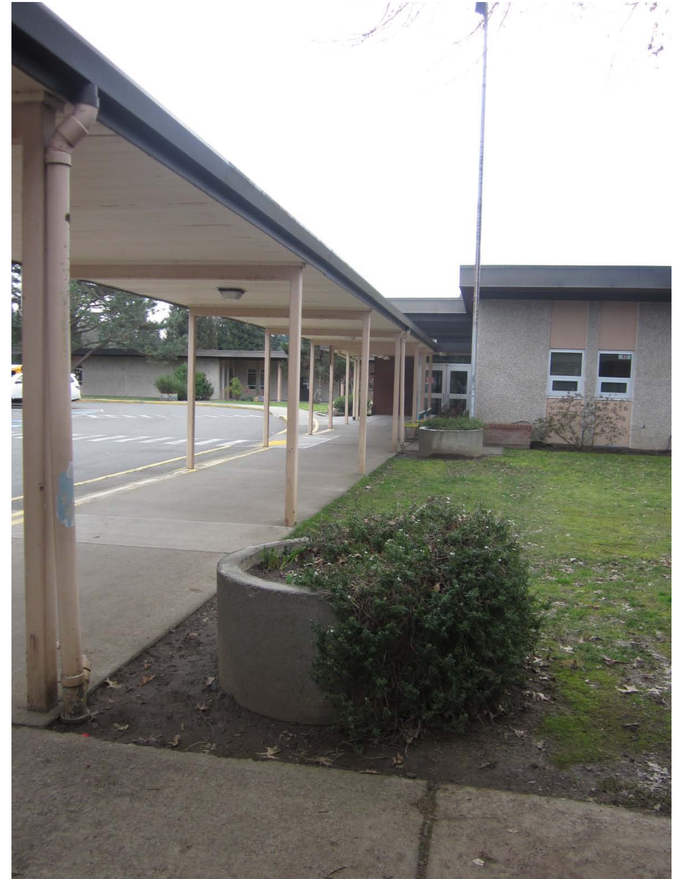
Front drop off, looking south
