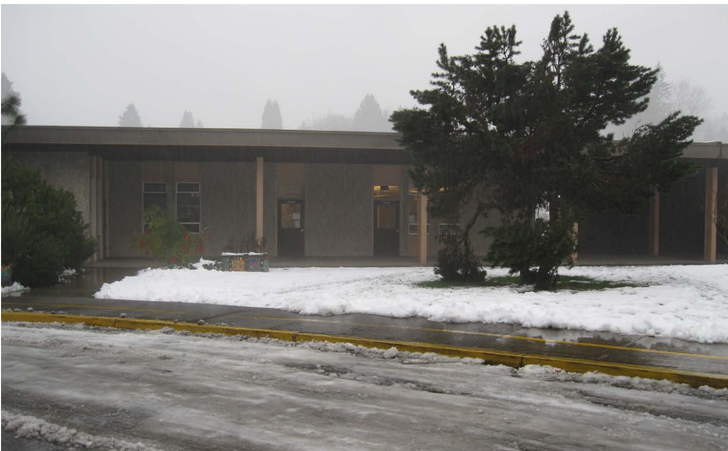
Classrooms near the front entry, looking south
