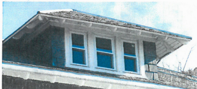
Hipped Dormer with Exposed Rafters
