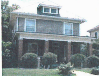
Combination of Brick and Shingle Siding
