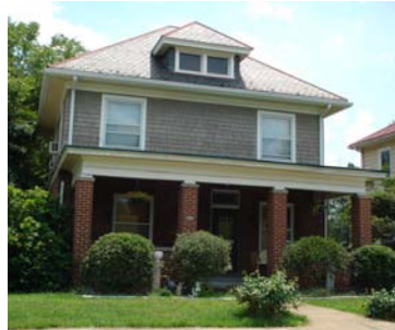
Combination of Brick and Shingle Siding
