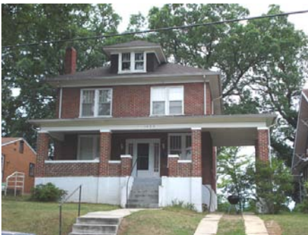
Porte-Cochere Accessed by Double Strips of Concrete
