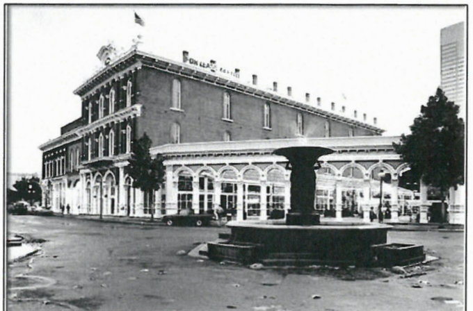
FIRST AVENUE - PORTLAND | CIRCA 1888 | CAST IRON COLUMNS
