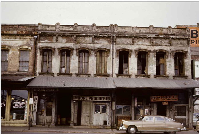
FRONT AVENUE - PORTLAND | CIRCA 1858 | CAST IRON COLUMNS & METAL AWNINGS
