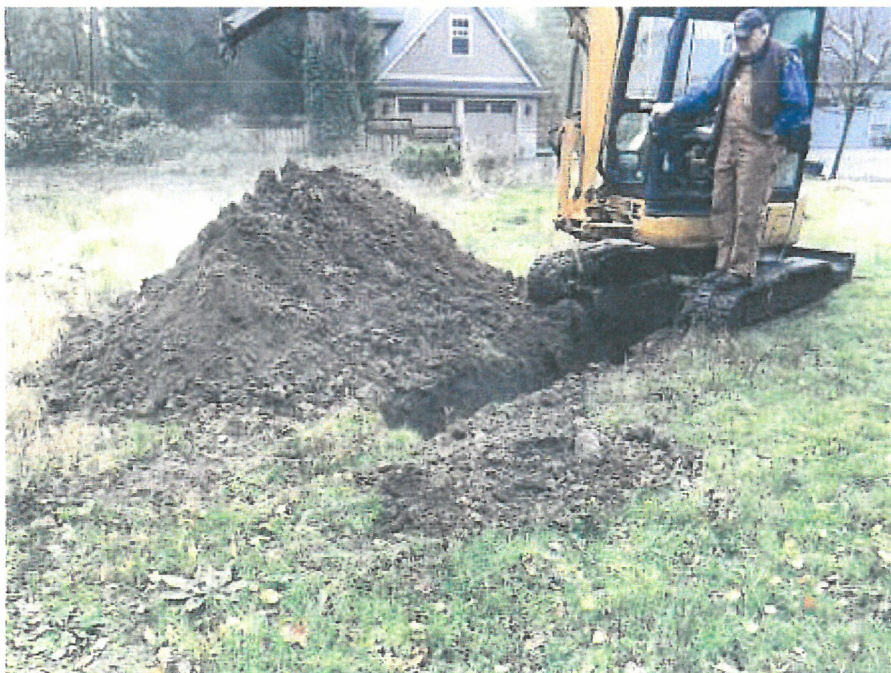
Test Pit TP-1
