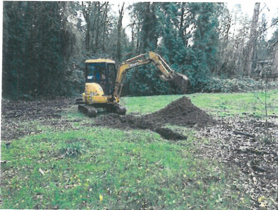
Test Pit TP-4
