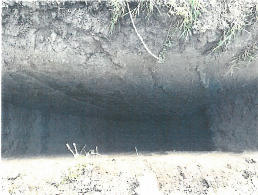
Test Pit TP-1
