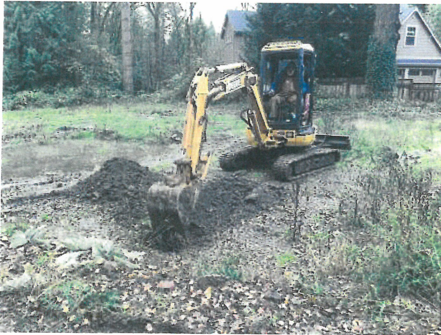
Test Pit TP-2
