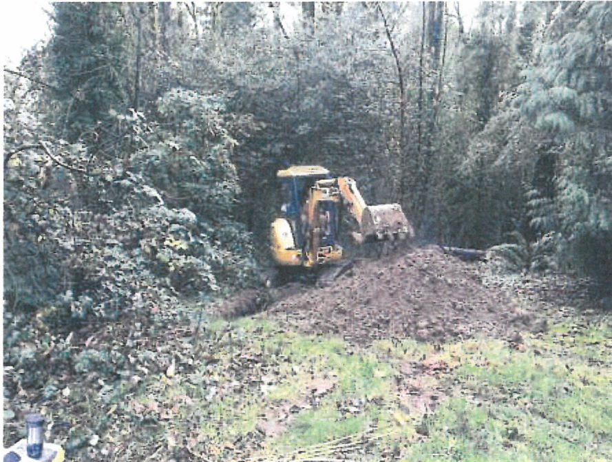
Test Pit TP-3
