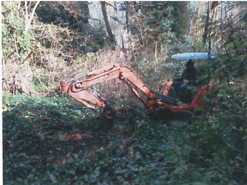
Test Pit TP-2
