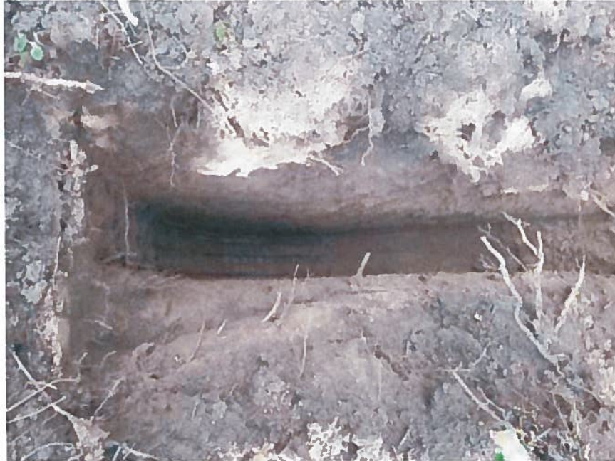
Test Pit TP-1
