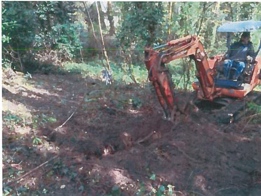
Test Pit TP-1
