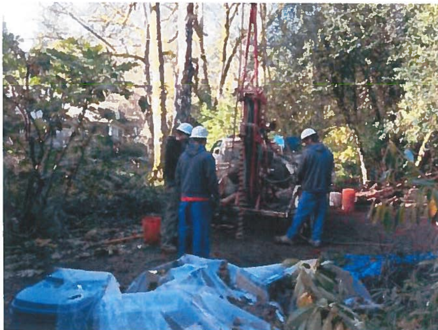
Drilling Soil Boring in Building Location
